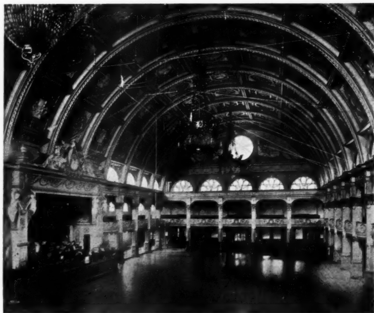
Blackpool Winter Gardens: The Ball Room. The floor is of oak boards in narrow widths. Bordering the floor is the dancers' promenade, above which is the spectators' gallery. The orchestra is on a dais on the left of the picture.
