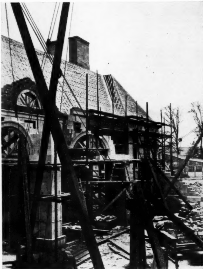
Figure one. Gledstone Hall in process of erection. The radial bed of a voussoir is being dressed to permit of the formation of joints of uniform width. Wooden casings protect the bases of columns and piers.
