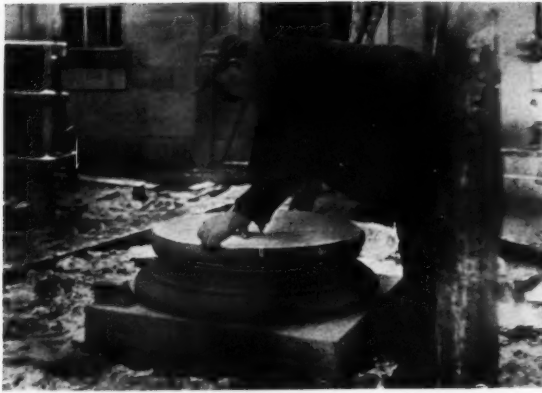
Left, figure five. Marking out the position of the drum on the base, which has been already set. The zinc template used for marking out the plan on the underside of the drum is used for establishing its future position on the base. Right, figure six. Planing the surfaces of a block of stone by machinery. A great number of different shapes can be produced by adjusting the relative positions of the block to the cutting edge, but the machine is most useful in the preparation of many blocks of similar shape.
