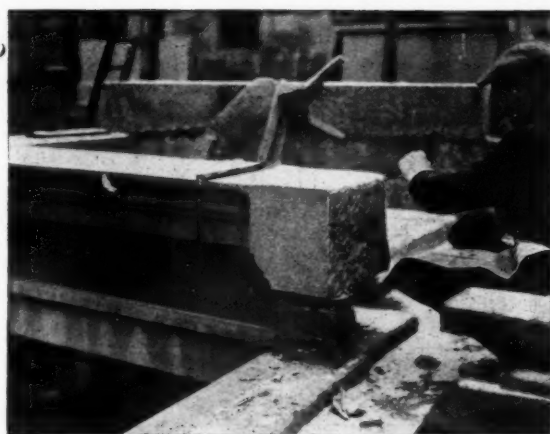
Left, figure two. A final paring away of a back edge to permit of uniform jointing. The mason is using a "mallet-headed" chisel, i.e. one provided with a swelled-out driving end. The small brick pier supports the cornice while it settles equally on its green mortar bed. Right, figure three. A large block in preparation for the lower drum of a column. The angles of the square have been pared away to form an octagon, whose angles are now being pared away to form a sixteen-sided prism. Convex and concave templates of zinc are used in marking and testing the curvature of the shaft.
