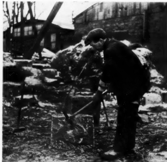
Figure seven. While the machine is in action in the shed, the old-fashioned pick is in operation outside. The lower portion of the stone surface has been already treated, and the degree of uniformity obtainable by the pick may be realized from its appearance.
