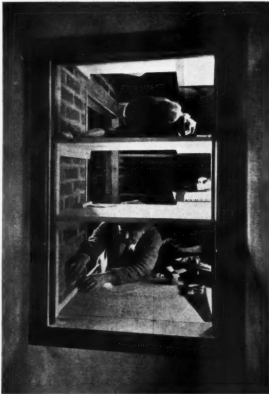
Figure three. Marking on a piece of moulding the pattern of the undulations of the slightly irregular surface of the wall against which it is to fit.
