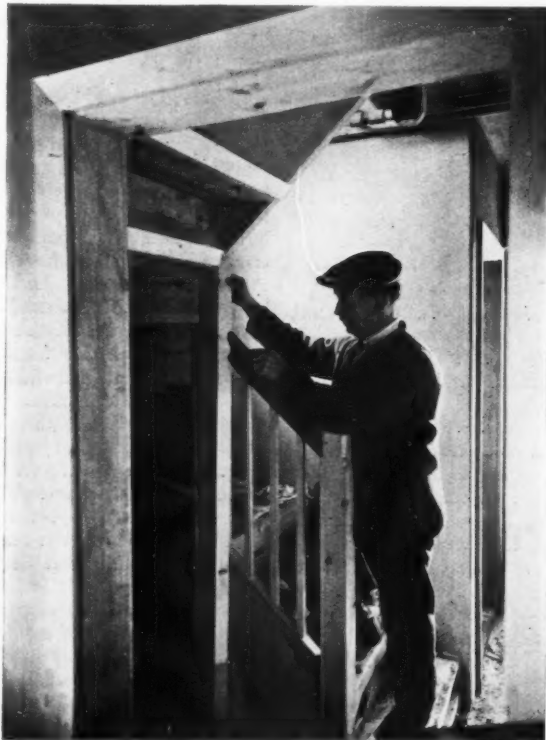
Figure one, left. Trying an architrave fillet in position after scribing it to fit the moulded hand-rail. The torus beads of the outer string have been notched to permit of this. Figure two, right. Stairs in process of being fitted. The grooves and wedges used for fixing the risers in the strings and the angle blocks below the treads are clearly seen.
