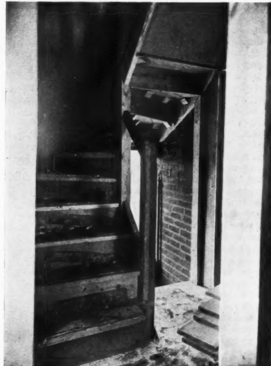
Figure one, left. Trying an architrave fillet in position after scribing it to fit the moulded hand-rail. The torus beads of the outer string have been notched to permit of this. Figure two, right. Stairs in process of being fitted. The grooves and wedges used for fixing the risers in the strings and the angle blocks below the treads are clearly seen.
