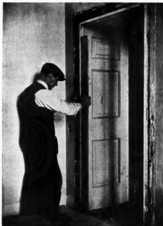
Left, figure five. Testing the paneled jamb lining for verticality. African mahogany has been used for the joinery, though the grain of the wood is hidden under the priming coat of paint. The tenons of the surrounding framed grounds are seen on the right. Right, figure six. Lighting and ventilating areas contrived in the roof of Gledstone Hall to serve the attic floor without intruding dormers in the outer roof slopes. Uniform close joints around the casements indicate the care exercised in their fitting.
