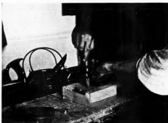
Figure four. Screwing and gluing the architrave into the plinth block. A bare-faced tenon has been formed on the architrave moulding, and a corresponding groove in the plinth block.
