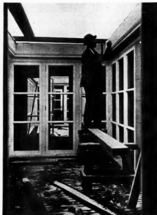
Left, figure five. Testing the paneled jamb lining for verticality. African mahogany has been used for the joinery, though the grain of the wood is hidden under the priming coat of paint. The tenons of the surrounding framed grounds are seen on the right. Right, figure six. Lighting and ventilating areas contrived in the roof of Gledstone Hall to serve the attic floor without intruding dormers in the outer roof slopes. Uniform close joints around the casements indicate the care exercised in their fitting.
