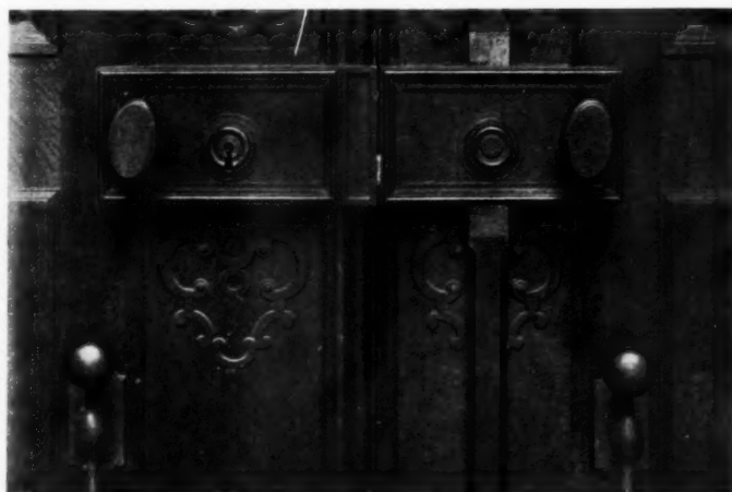
Combined mortice lock and espagnolette by Bagues, Ltd.
