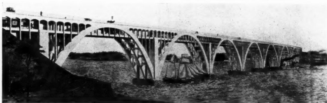
Bridge over the little belt, Denmark. By Jultent and Fyn. In this design for a reinforced concrete bridge a series of arches follow the main pattern of the structure, while all the other members of the framework are either vertical or horizontal.
