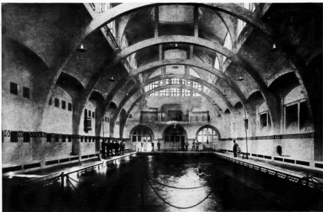
Figure nine. The reinforced concrete swimming-bath recently erected in Paris is unusual in treatment, and shows a more imaginative use of the material than is usually to be found in this country. There are no dressing-boxes.
