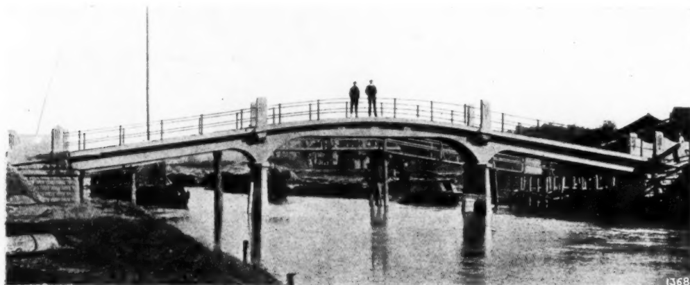
Pootung Bridge, Shanghai. A typical example of the traditional footbridge in reinforced concrete. A feeling of restlessness is conveyed by the fact that the central span does not follow the line of the footway.
