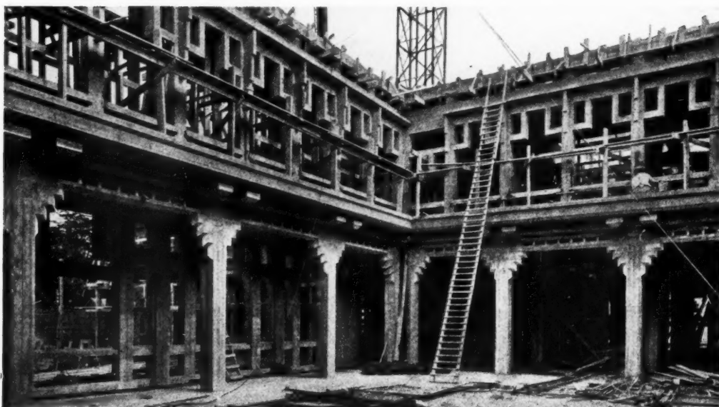
De Nederlanden: a modern office block at The Hague. By H. P. Berlage. This building is a very important experiment, because it shows evidence of a desire to profit from the vast experience in "post and beam" design which is embodied in the wooden buildings of China and Japan. The framework is composed in a pattern having rectangular subdivisions, and so is aesthetically related to the horizontal and vertical lines of the building itself.
