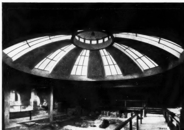
The covering to the Kingston baths at Bath. By Alfred J. Taylor. The dome is 35 ft. in diameter, with a rise of 10 ft. The lantern and the ribs of the dome are of reinforced concrete. Above, an interior view. Below, plan and sections.
