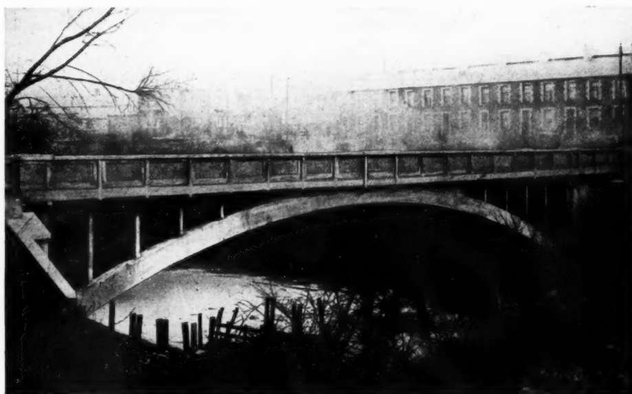
Abercynon Bridge. This has a span of 130 ft., and the radius of the arch is 156 ft. 8 in. The footways are cantilevered out from the main body of the structure.
