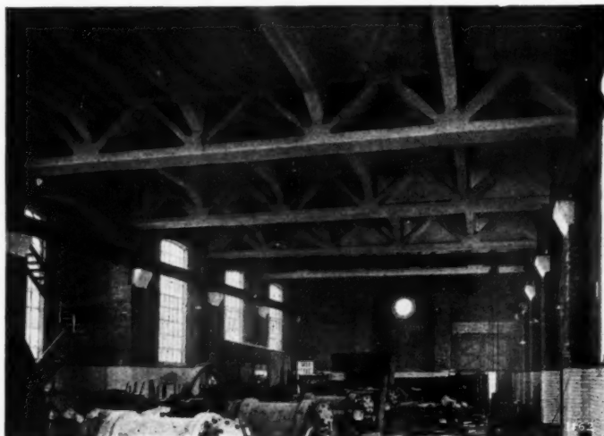
Refrigerating station for the Port of London Authority. Here the constructional members which support the ceiling are composed of framework of a pattern consisting of a series of triangular shapes. These are in themselves quite orderly, and as they are enclosed within long rectangles, having their sides parallel to the wall and to the floor respectively, they are well subordinated to the surrounding architecture.
