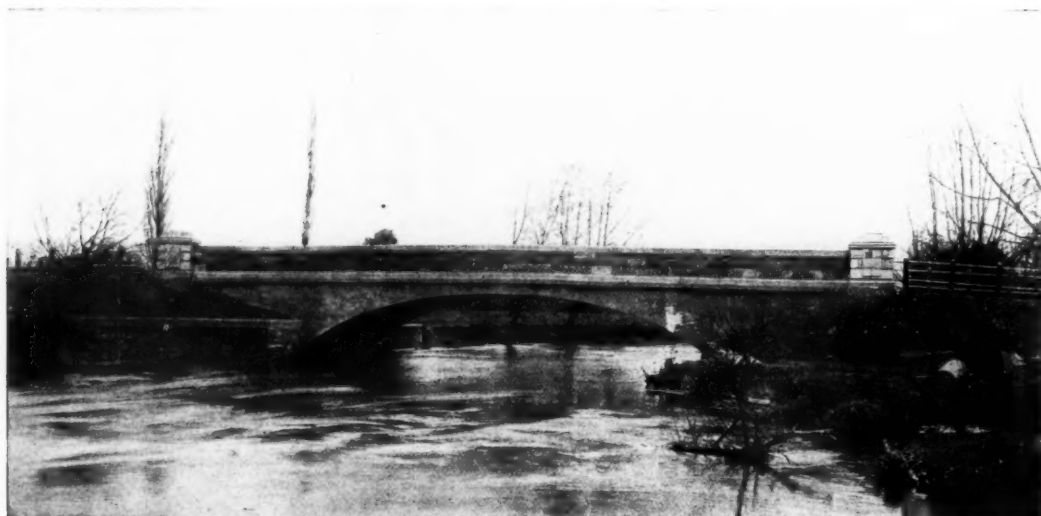
Weegin's Bridge, Herefordshire. An example of a concrete structure based upon traditional masonry design, with spandrels unpierced.
