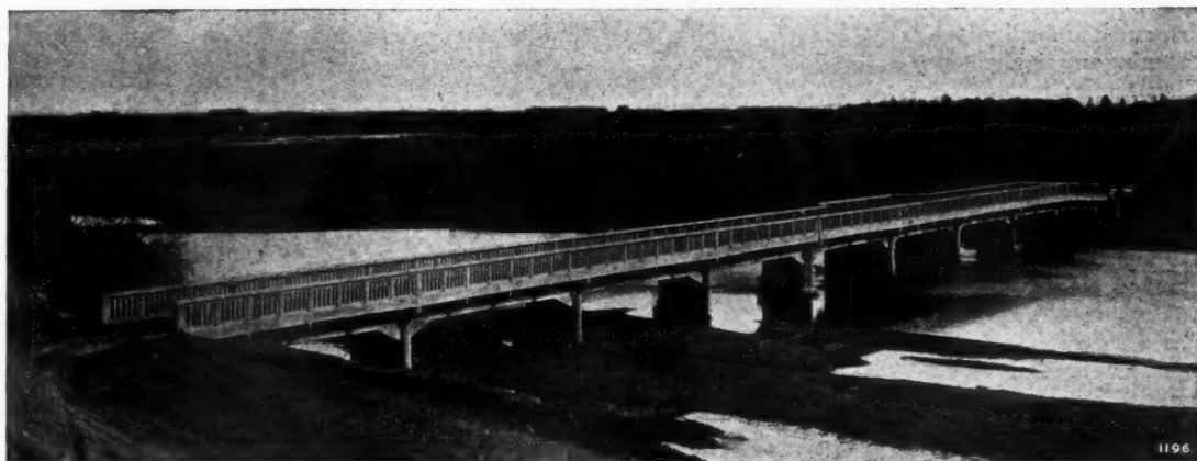
The bridge at Waipurkarau Gorge. It is 360 ft. long, and has nine spans of 40 ft. each. A suggestion of timber construction is noticeable, although the bridge is actually of reinforced concrete.
