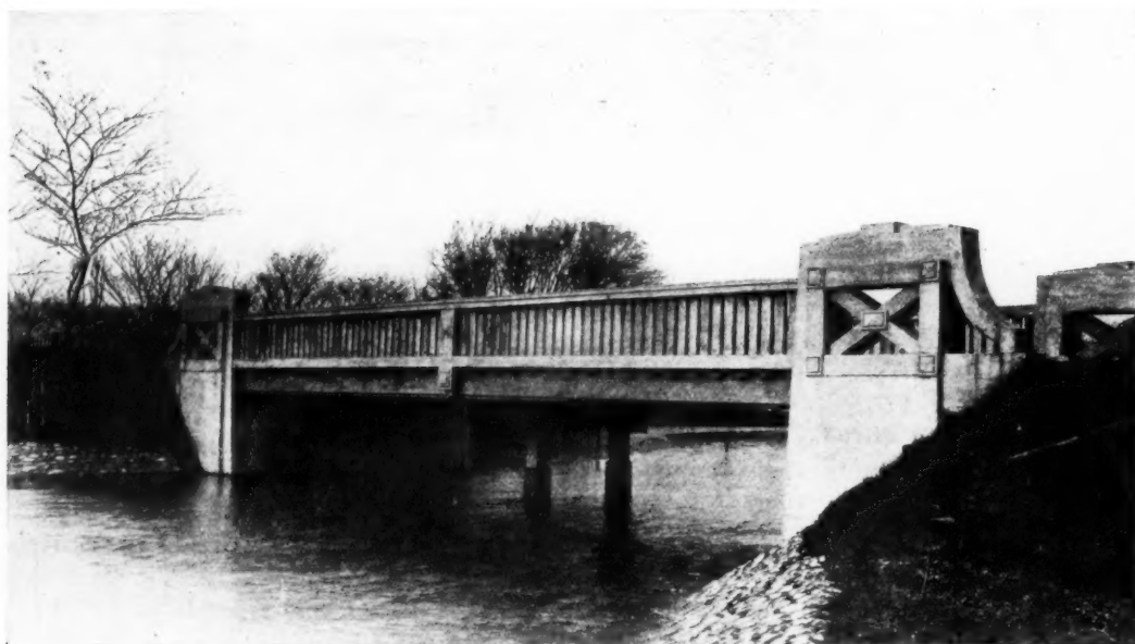
This bridge at Barrow-in-Furness is strongly reminiscent of timber construction in its actual span, whereas the treatment of the abutments is one which is only possible in concrete.
