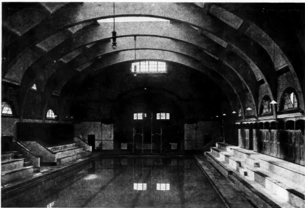
Figure eight. The bold reinforced concrete ribs, elliptical in form, which are thrown across the hall, are features in this design, in which the amphitheatre system of seating with dressing-boxes planned at a higher level is also adopted.
