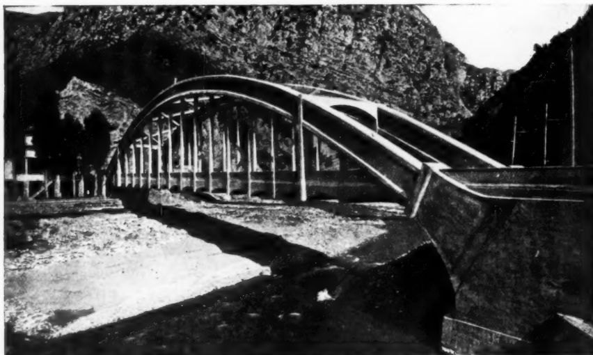
A bowstring bridge over the Vesubie River. It has a span of 315 ft., and is constructed with temporary hinge joints, filled in after the structure had taken up its permanent position.
