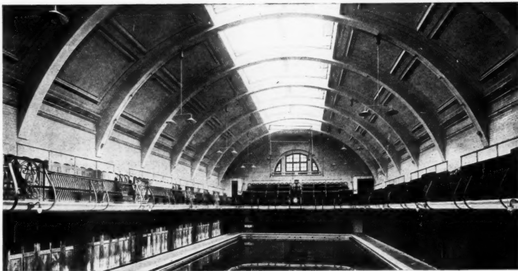
Figure eleven. Bath at Hammersmith. By J. E. Franck. The orthodox arrangement of dressing-boxes under an overhanging gallery is here followed. Special attention has been given to the excellent design of the top-lighted bath hall.
