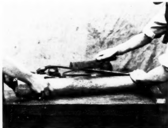
Left, figure three, a further stage in the pipe-bending operations. Hauling snatch bobbins through the partly bent pipe by means of sashline and a plumber's hammer. Right, figure four, bending the pipe. Dressing down the bulges formed in the lead by the action of the dummy. A boxwood dresser is used for this purpose in the final stages, and beech or hornbeam dressers during the roughing out.
