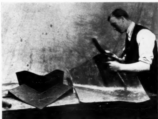
Left, figure one, commencing the formation of an "internal break" with the bossing-mallet in the left hand and the bossing-stick in the right. The shears or "snips" are in the background, and the handle of the boxwood "dresser" is seen on the extreme left. Right, figure two, starting to make a "square bend" by first kinking the pipe and then smoothing out the kink with the dummy. These dummies have iron handles and heads of plumber's solder wiped on to screw sockets.
