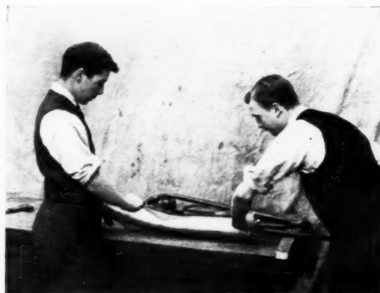
Left, figure one, commencing the formation of an "internal break" with the bossing-mallet in the left hand and the bossing-stick in the right. The shears or "snips" are in the background, and the handle of the boxwood "dresser" is seen on the extreme left. Right, figure two, starting to make a "square bend" by first kinking the pipe and then smoothing out the kink with the dummy. These dummies have iron handles and heads of plumber's solder wiped on to screw sockets.
