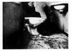
Left, figure two. Plumber at work in a small house soldering in the brass grid to the waste from a bathtray. The modern use of galvanized from pipes with lead branches is also illustrated. Right, figure three. Packing the crack of the joint between a brass collar and the stoneware outlet with a ring of twisted newspaper to prevent the cement oozing into the bore of the pipe and obstructing the flow.
