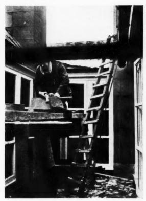
Left, figure five. Preventing the accumulation of greasy splashes in the crack between a sink and the adjoining cupboard. The strip of lead is close copper-nailed on the wood and dressed over the stoneware. Right, figure six. Plumber at work in an internal area at Gledstone Hall. Bossing-up an internal break from a piece of sheet lead.
