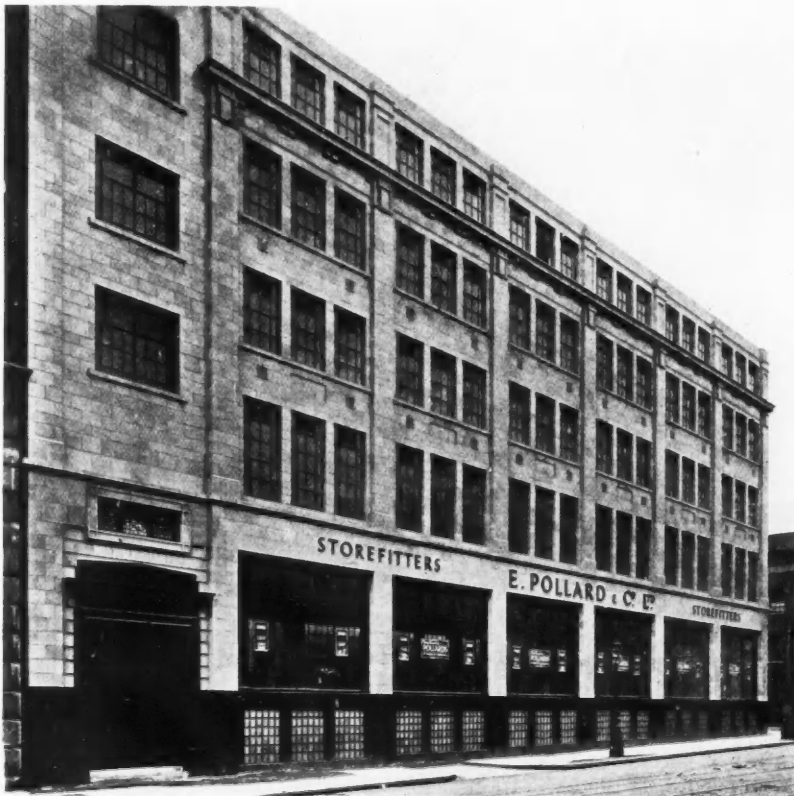
Messrs. Pollard's new joinery works, Clerkenwell, E.C. By Malcolm W. Matts. Above, a board-room in Italian walnut. Below, the main front. The building is of steel-frame construction with reinforced concrete floors. The exterior is of cream faience with a base of black granite.
