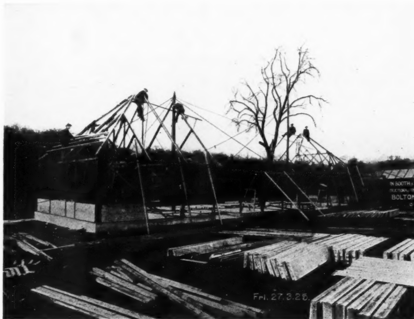
Bungalows at Nottingham. By T. Cecil Howitt. The erection of the framework.
