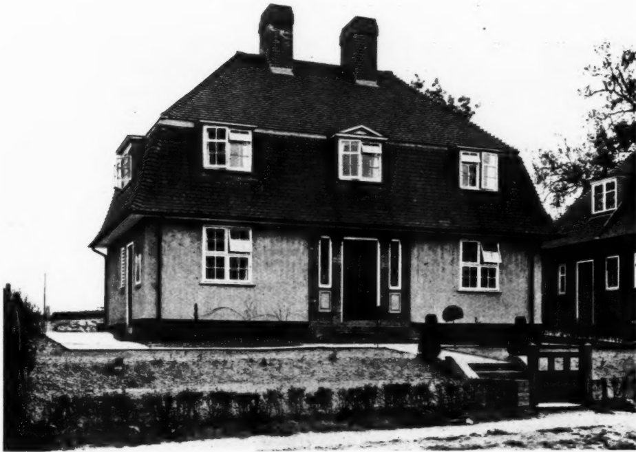
44 Northway, Hampstead Garden Suburb. By C. G. Butler. This house is the centre one of a group of three, those on either side being of a semi-bungalow type. The walls are treated with smooth stucco finished cream colour, the plinth is tarred, and the tiles for the mansard roofs are similar to those described on the opposite page. Above, a view facing north. Below, the ground-floor plan.
