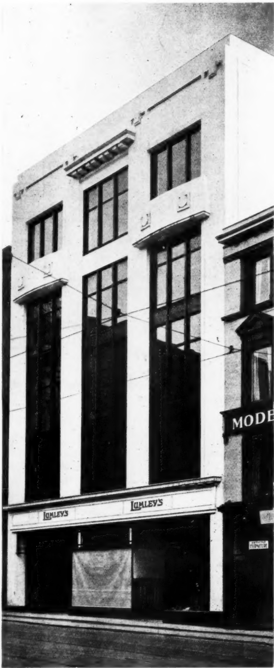
Messrs. Lumley's premises in Sauchiehall Street, Glasgow, illustrated above, were formerly a cinema house. The conversion and reconstruction are the work of William Inglis and Thomas Ramsay. The front is of brick finished with a proprietary plastic material.
