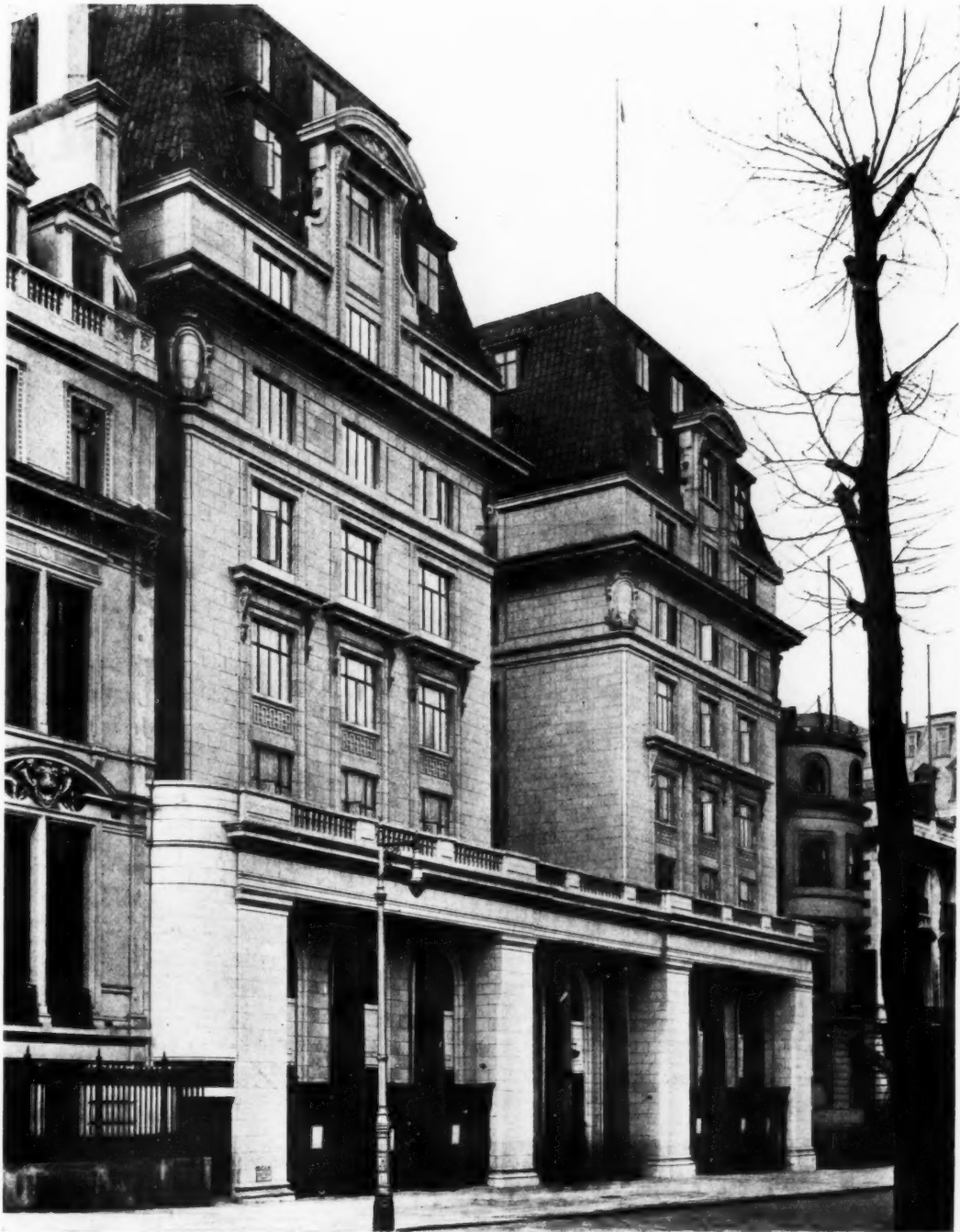
Park Lane Hotel, London. By Messrs. Henry Tanner. Of steel-frame construction, the building was commenced in 1913, but the work was stopped a year later and not resumed till the autumn of 1925. The completion of the structure, which is faced with matt-surfaced ivory-tinted terra-cotta, involved important alterations to the original steelwork. Fire-resisting floors and roofs have been employed throughout the building, and every bedroom in the hotel has its own private bathroom. Above, the Piccadilly front.
