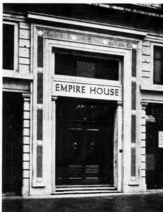
Empire House, St. Martin's-le-Grand, London. By Gunton and Gunton. Above, the principal entrance showing the solid bronze outer doors. Below, the entrance hall. This is lined to the full height of the walls with Ashburton and Petilor marbles, and paved with large unpolished squares of Hopton Wood stone.
