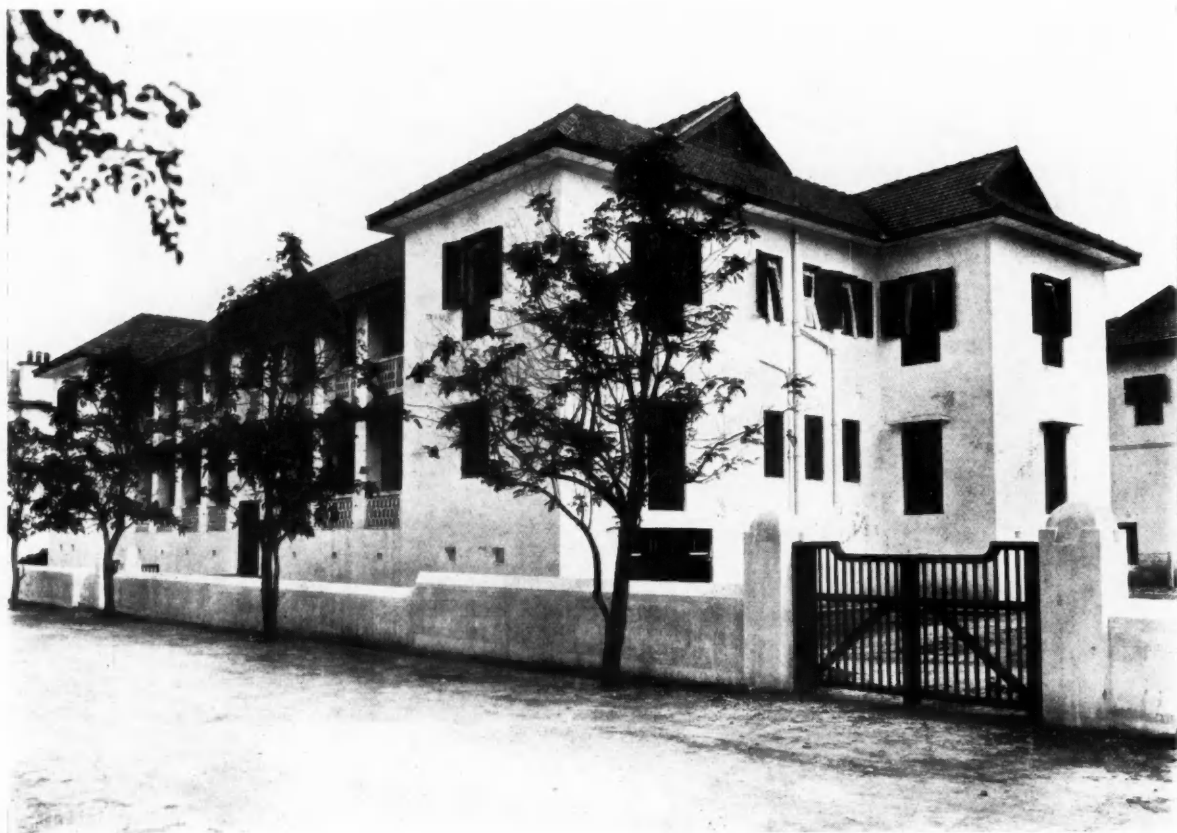
A block of four flats in Zanzibar. By P. C. Harris. These sun-excluding flats were recently erected by the Public Works Department for the occupation of Europeans, and are planned to secure the full benefit of the north-east and south-west monsoons. The walls are of coral rag, plastered externally and internally; the roofs are covered with Mangalore red tiles; and the veranda rails and "ghallis" are cast in white Portland cement. Above, a general view. Below, the plans, which are reproduced to a scale of \frac{1}{32} in. to 1 ft.
