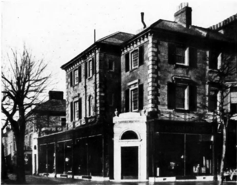
Above, Messrs. Charringtons' coal order offices at Romford, Essex. By John Seely and Paul Paget. The building has been entirely re-modelled, the work including the simplification of the gable copings and chimney-stack and the insertion of new windows and a door. The brickwork is lime-whited and the door and window heads are of red roofing tiles laid on edge. Below, new shop premises to No. 11 Cornfield Road, Eastbourne. By B. Stevens. The shops are well lighted, and are approached from the wrought-stone entrance doorway at the junction of the two frontages.
