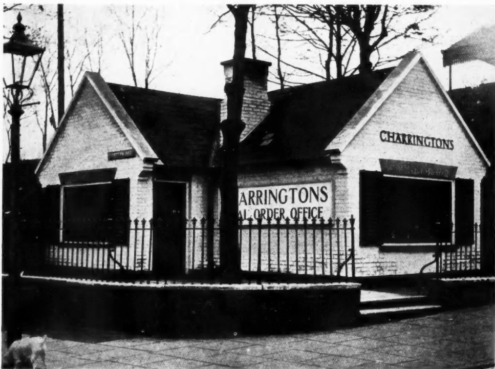
Above, Messrs. Charringtons' coal order offices at Romford, Essex. By John Seely and Paul Paget. The building has been entirely re-modelled, the work including the simplification of the gable copings and chimney-stack and the insertion of new windows and a door. The brickwork is lime-whited and the door and window heads are of red roofing tiles laid on edge. Below, new shop premises to No. 11 Cornfield Road, Eastbourne. By B. Stevens. The shops are well lighted, and are approached from the wrought-stone entrance doorway at the junction of the two frontages.
