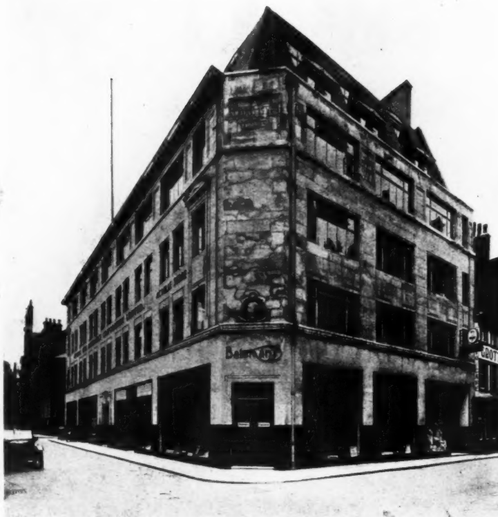
Above, Daniel Neal and Sons, Kensington High Street, W. By P. J. Westwood and Emberton. An example of the arcaded front which is being widely adopted throughout Great Britain. A long span of fascia is boldly supported by columns, and the central windows have given place to showcases which provide a greater area for the display of goods.
