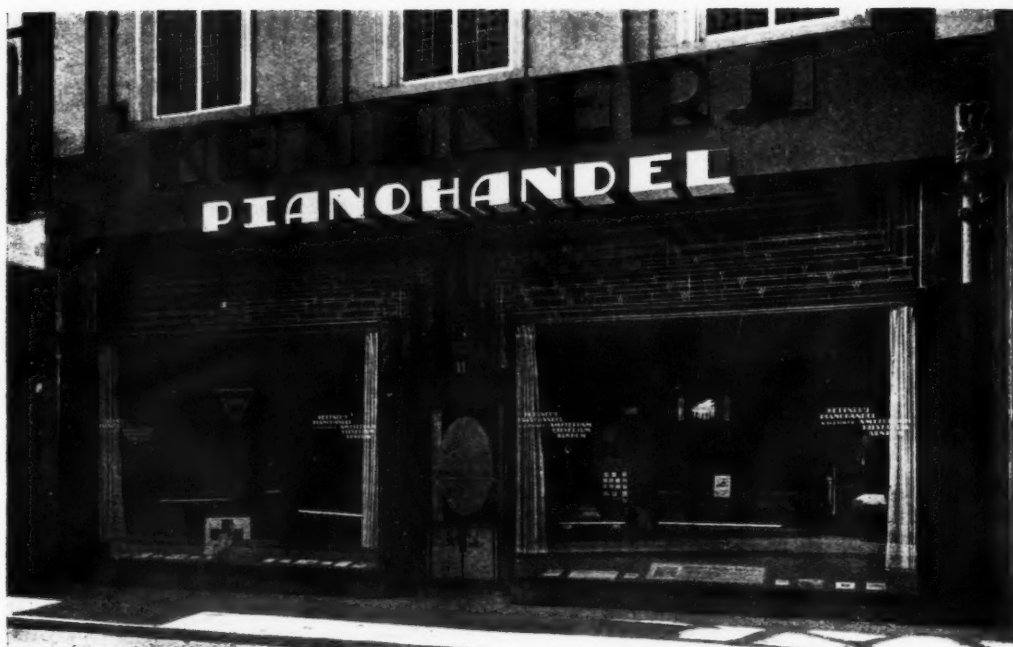
Kettners' Pianohandel, Utrecht. By J. F. Staal. The fascia lettering is most successful in its handling, and certainly original. In order to give a deep soffit to this lettered fascia, without loss to floor space below, the upper part of the shop window has been designed in recessed planes. This solution of the problem is rather more original than successful. The entrance doorway appears to suffer considerably from the treatment, and it does not appear to have sufficient space allotted to it.
