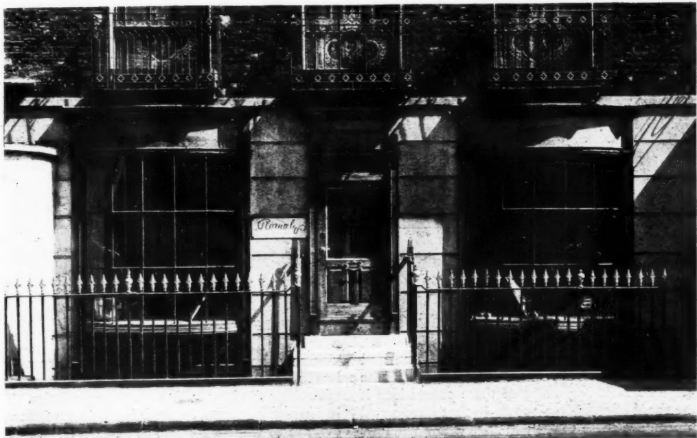
This firm in Beauchamp Place, S.W., too reticent to state its business, is well served by this delicate and restrained front, which has been contrived at the base of an early nineteenth-century terrace house. The detail of the wood pilasters and entablature to the door and windows is chastely classic, and the small-paned glazing appropriate to that of the windows over. Deep fascias, in conjunction with shadow from the balconies, minimize any effect of weakness induced by enlargement of the ground-floor openings.
