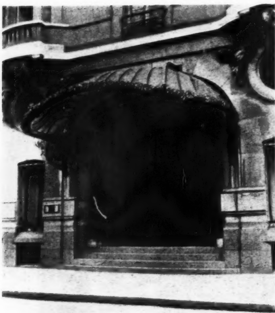
This marquee marks the entrance to an hotel in the Boulevard Raspail, Paris. Apart from being an exceedingly rich example of wrought ironwork, it is a remarkable study in solid geometry. Each glazing bar is curved in three dimensions, and no two squares of glass are alike. The support of the marquee is effected by the small brackets on either side, and by curved cantilevers from above, from which the outer frame is suspended.
