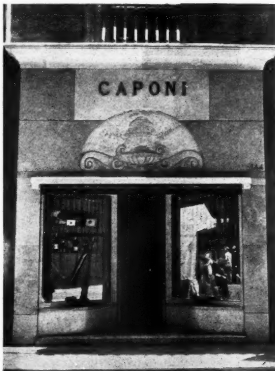
A confectioner's shop in the Corso Umberto, Rome. By Vinallia. The stone of which this succulent-looking little shop front is constructed is fawn-coloured, and is finished in a medium polish. The lunette of soft white stone has the lightness of a meringue. Note the peculiar window-boxes. Each contains a single box plant.
