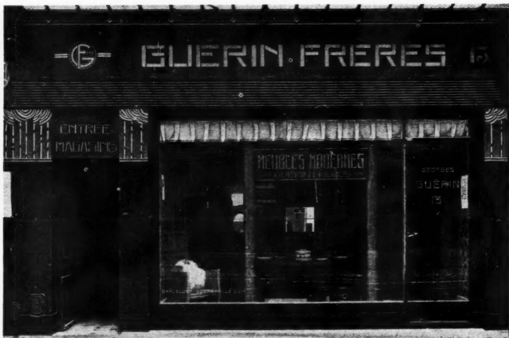
Guérin Frères, Rue du Faubourg St. Antoine, Paris. By Coudyser. This shop front is carried out in oak, tinted in various colours. The material is highly appropriate to the furnishing firm whose goods it displays. No transoms or stallboards obstruct the view of the large-scale articles exposed. The reeded architrave below the fascia is very effective as a continuous frame. The carved and painted pilasters are refreshingly original, and together with the lettering suggest a highly modern type of furniture within. The continuity of the glass area is not even broken into by the doorway, which is of noticeable simplicity. Here the whole shop itself becomes a showcase.
