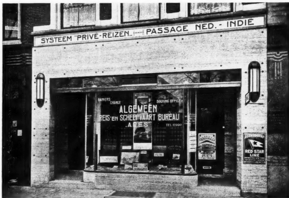
The office of a steamship agent at The Hague, Holland. By F. de Bruijne. The slabs of travertine of which the surround is made up are bolted through in the fashion inaugurated by the Viennese school of modernist designers. The deep stone architrave has been left unencumbered with lettering, the latter being relegated to a comparatively narrow strip above it. The window between the two entrances has been frankly treated as a showcase.
