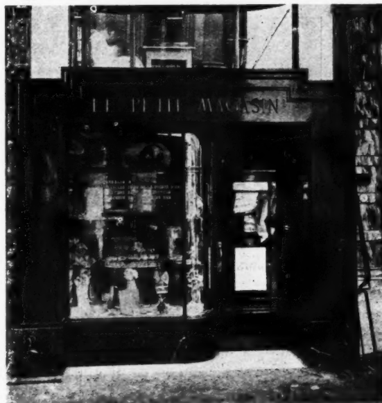
Le Petit Magasin. A men's shop in the Place de Brouckère, Brussels. By Frederick Sage. This façade, which is by a Belgian designer, shows a door deeply recessed, with a single window rounded back to it, and glazed without bars except for an angle vertical and a horizontal at frieze level, picking up the line of the door-head. The exceedingly heavy, moulded frame which surrounds door and window is successful in isolating them; over is a mezzanine window with a plain margin and similarly unbroken glazing.
