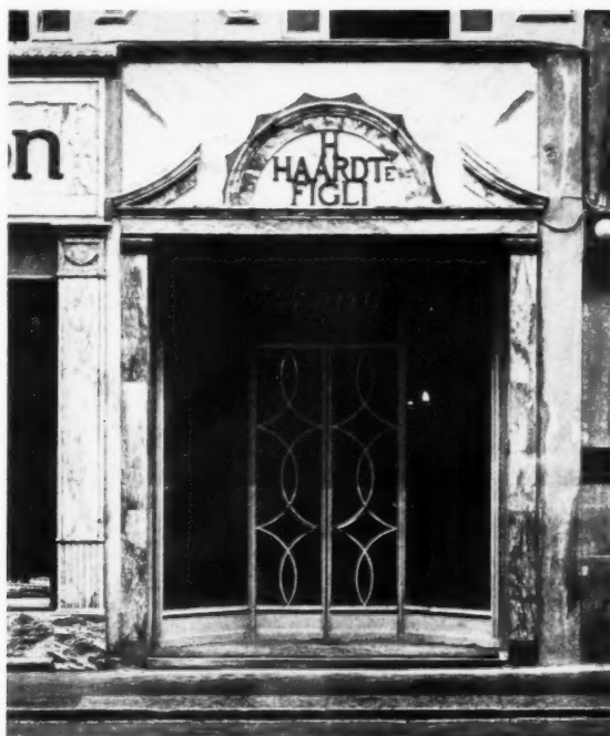
In this exquisite little draper's shop front in the Corso Vittorio Emanuele, Milan (by Dr. Giulio Magistretti), two kinds of marble have been used. The framework of jambs, architrave, broken pediment, and suspended archivolt are of Siena marble, while the background is formed of veined Serravezza. The handles to the entrance doors, which follow the curve of the glazing-bars, should be particularly noted.
