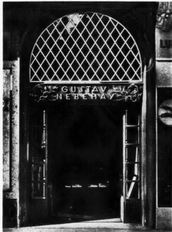
Gustav Nebehay, Vienna. By Professor Josef Hoffmann. The treatment of this entrance is comparable with that of the Chemiserie Gilmondré, which is illustrated below. The sides of the doorway itself are lined with showcases, which attract the notice of the passer-by without seriously incommoding the width of the entrance.
