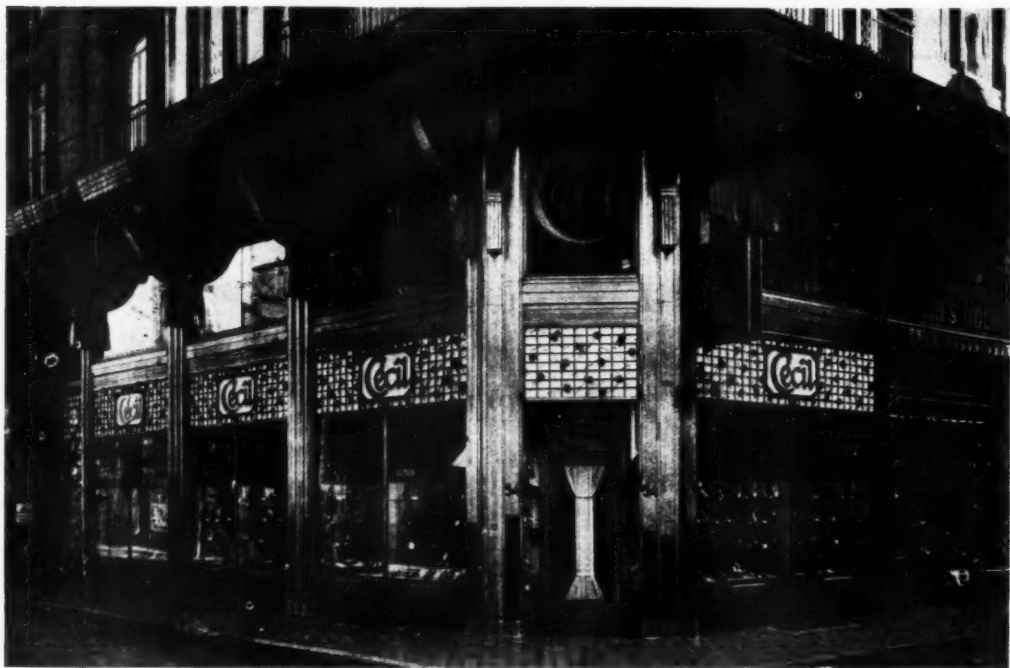
Shoe shop in the Rue Neuve, Brussels. By M. Kielbaye. This shop possesses a light and fanciful note. It exemplifies also the fact that metal imposes naturally a vertical treatment, having entirely different proportions from a marble frame. The upper façade is well separated and supported by the strong projecting balcony with its scalloped fascia and shaped brackets. Marble is here used as a base, though perhaps bronze would have better maintained the consistency of the treatment. The clustered metal columns nicely hold the balance between lightness of effect and structural strength. The decorative motif in the fanlights should be compared to the simplicity of the corresponding feature in the Chaussures Raoul, Paris (page 863).
