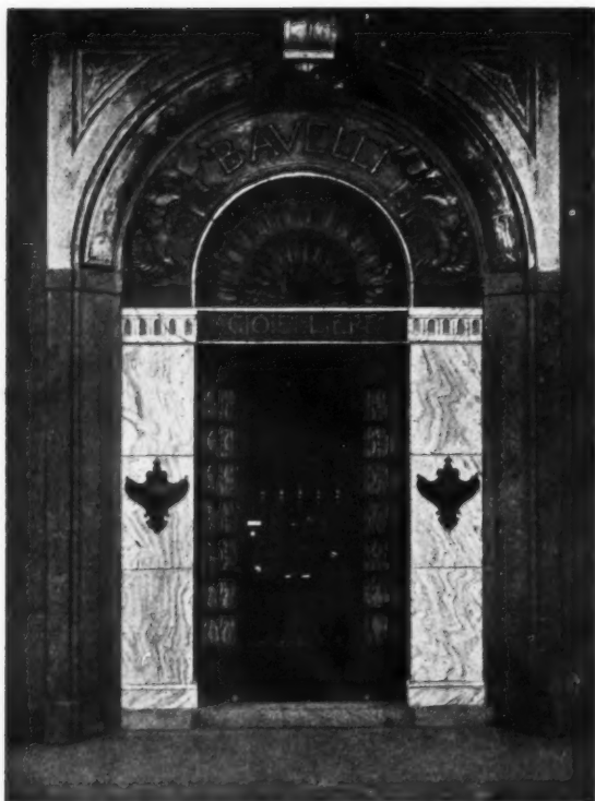
A jeweller's shop front in the Piazza di S. Giuseppe, Milan. The jambs are built up of large slabs of Cipollino marble. The door and fanlight are of bronze and wrought iron, the latter being set in a surround of beaten copper. The lintel on which the business of the firm is described is also of copper.
