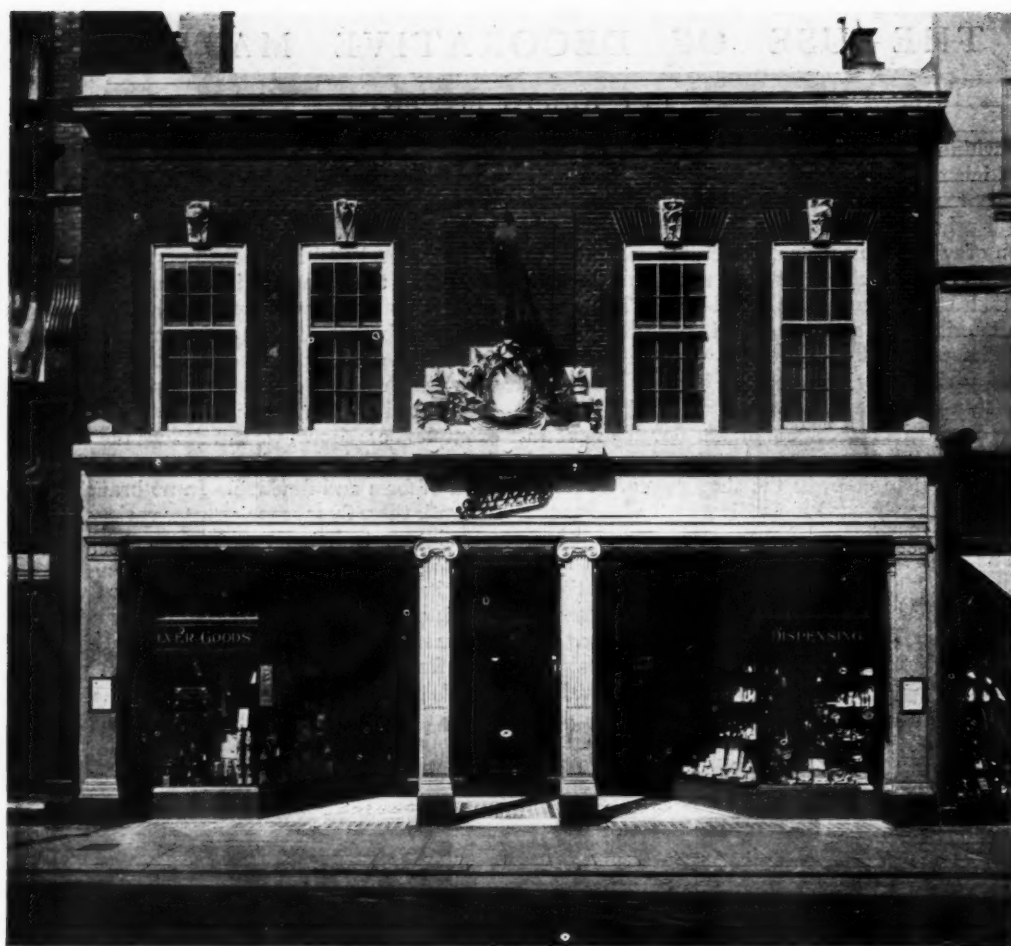
Boots' Shop, Palmerston Road, Southsea. By F. W. Gregory. The shop front here illustrated is carried out in silver-white granite pilasters and fascia, with royal-blue granite plinths, the shop framework being in teak and bronze, the upper part in 2 in. hand-made, sand-faced bricks, and Portland stone carving and cornice. Messrs. Boots must be congratulated on the distinctive architectural effect here obtained by the judicious employment of English traditional motifs. The arrangement of the recessed front is well conceived, with its dual entrance for circulation and inspection of goods. The Greek Ionic of the eighteenth-century apothecary is here utilized with excellent effect. With regard to the general composition, the feeling of duality, generally to be avoided, is produced by the close spacing of pilasters below and the solid panel above. A central window would have unified the composition in a more successful way.
