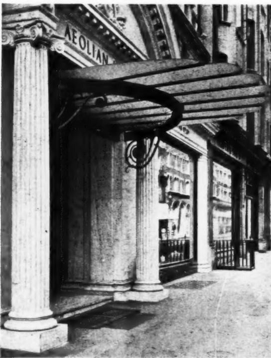
The Aeolian Hall, Bond Street, W. By E. Young, in collaboration with K. A. Braden. This marble entrance-way was not designed to take a marquee. The subsequent introduction of the latter was not, therefore, an easy problem. The maximum amount of projection over the pavement has been arranged, while the metal-work has been kept well back.
