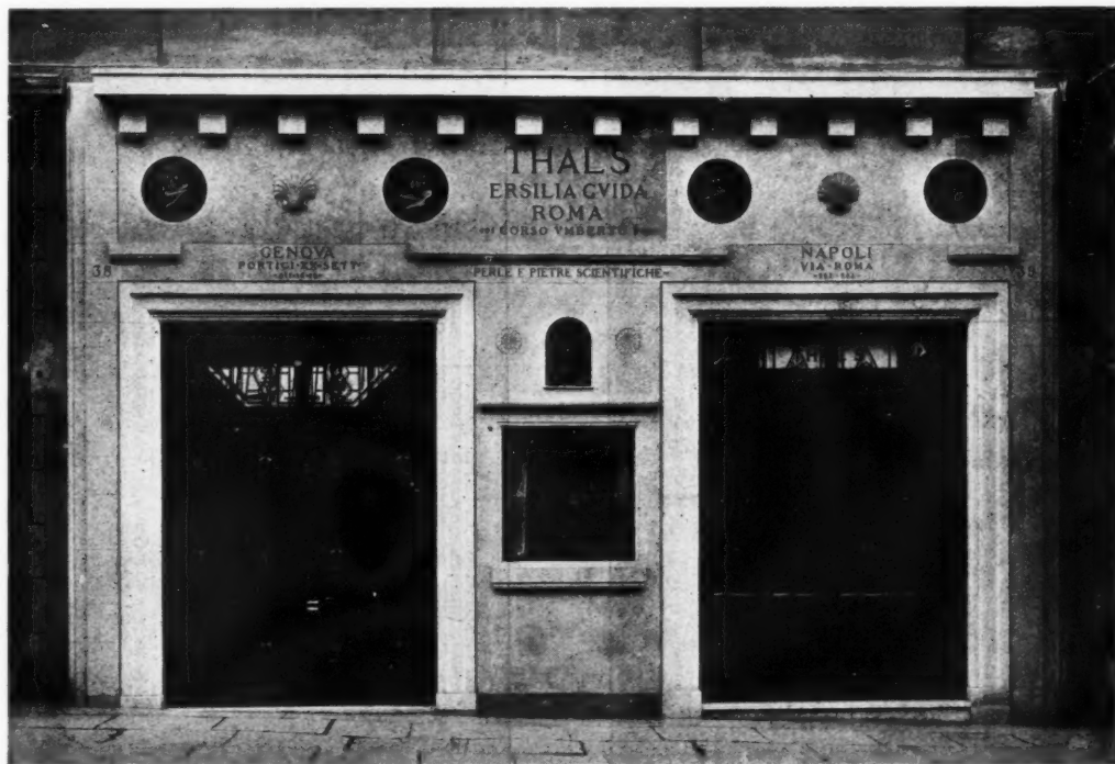
This jeweller's shop, in the Via Nazionale, Rome, by Arnaldo Fossini, is executed entirely in travertine, with plaques in bronze and window grilles in bronze and wrought iron, the metal contrasting strongly in both tone and texture with the light, plain surfaces of the marble. The precious quality of the goods to be sold is stressed in this shop front by an essentially secret character expressed especially in the close infilling of the windows. The lettering is well designed and disposed. In the lower illustration the centre showcase is empty, and the wrought-iron and bronze gates are closed over the larger window and entrance.
