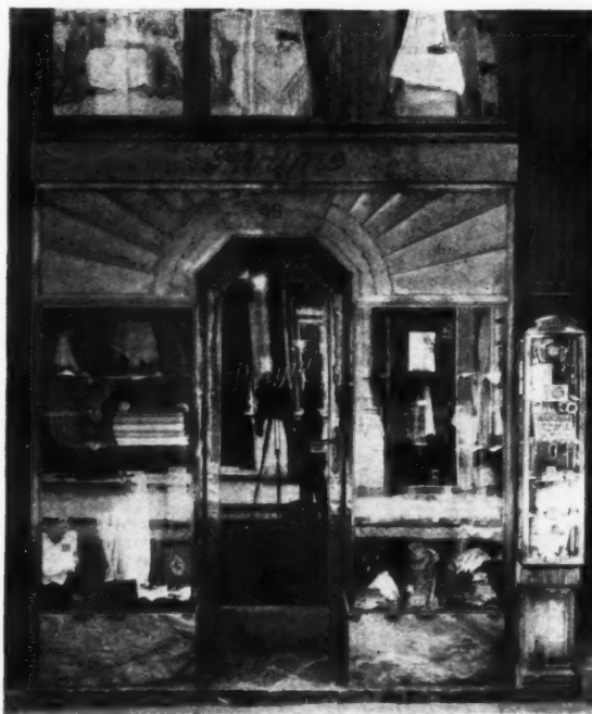
Phryné, Rue du Pont Neuf, Brussels. By Frederick Sage. This is a light metal shop front treatment in two stories, which relies entirely upon the delicacy of its proportions and composition for effect. No attempt is made to obtain, in such a narrow frontage, any special continuous surround.
