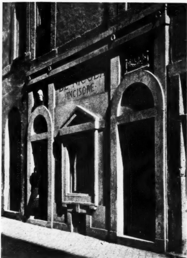
De Nicola, Rome. By E. del Debbio. This façade, for an engraver and stampcutter, in the very narrow Via Vittoria, Rome, is, like other Italian examples illustrated, of marble, the material being travertine and the treatment a simplified classic.
