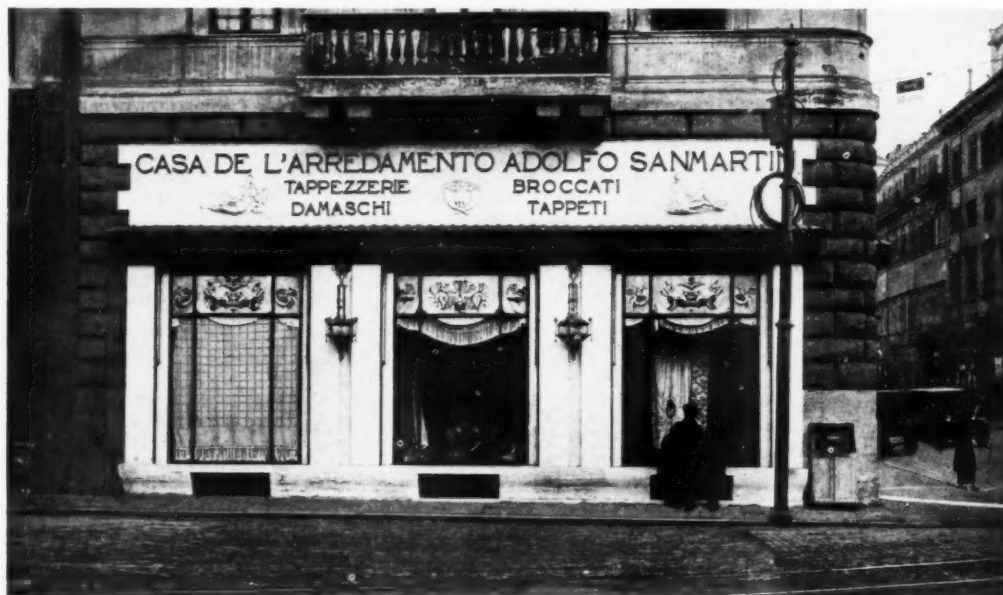
This Italian decorator's shop in the Corso Vittorio Emanuele, Rome (by Marcello Piacentini), shows how curiously neglected the pelmets are in England. Nowhere can one find any here with such carefully designed decorations. The masonry surround is of light-coloured Subiaco stone, with a wooden architrave.
