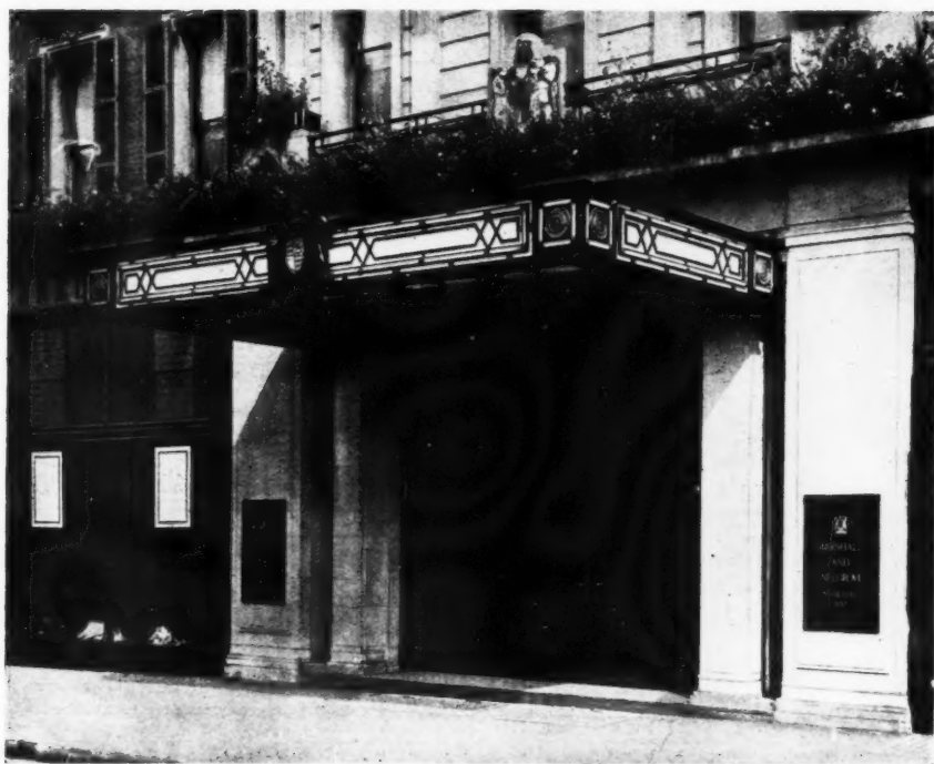
Marshall and Snelgrove, Oxford Street, London. By Gibson and Gordon. This marquee is familiar to Londoners in Oxford Street. It has been carried out in glass and coloured enamelled bronze. Unlike many others, it projects completely at right angles to the façade. Any apparent tendency to fall on the pedestrians beneath is negatived by its lightness of treatment. The metal work is kept to thin decorative dimensions only. The opaque glass and coloured enamels complete this sense of lightness and provide very decorative quality.
