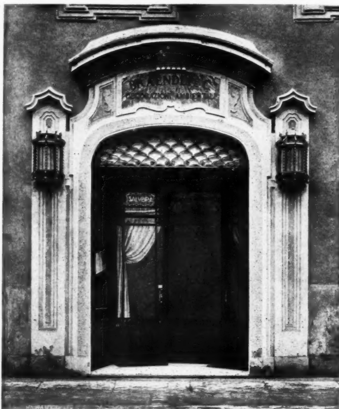
A jeweller's shop front in the Piazza di S. Giuseppe, Milan. The jambs are built up of large slabs of Cipollino marble. The door and fanlight are of bronze and wrought iron, the latter being set in a surround of beaten copper. The lintel on which the business of the firm is described is also of copper.
