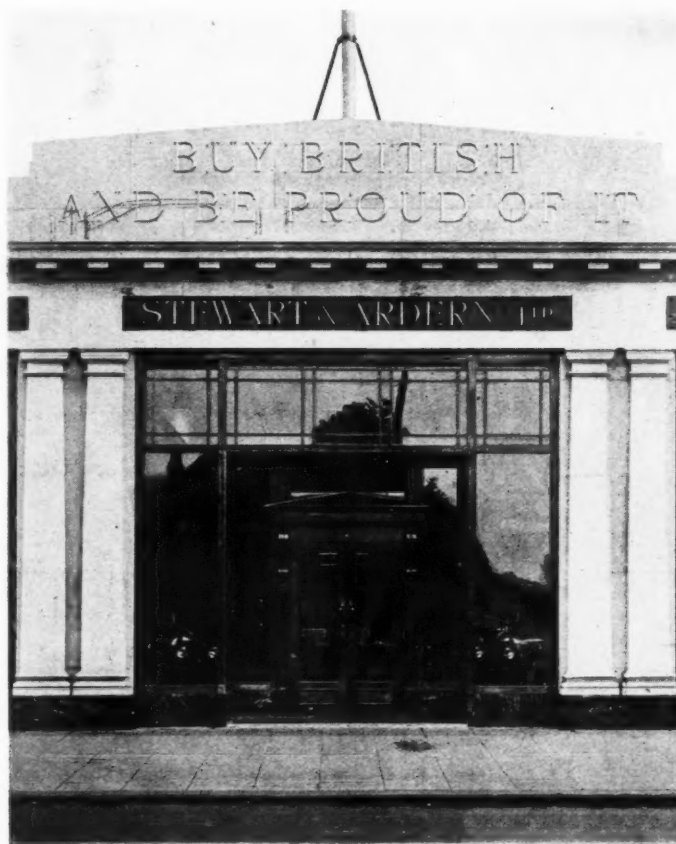
Stewart and Arden, Ltd. By Arthur H. Davis and Partners. This front has an eminently sane and straightforward appearance, and the combination of stonework, marble base, and bronze framework and door is well thought out. The lettering in the fascia is striking and yet in scale; but a more monumental effect would have been obtained by simply incising it in stone (see Austin Reed, page 861). The applied pilasters are, perhaps, a rather weak feature of the design, and the scale of the whole would have been greatly improved by their modification.
