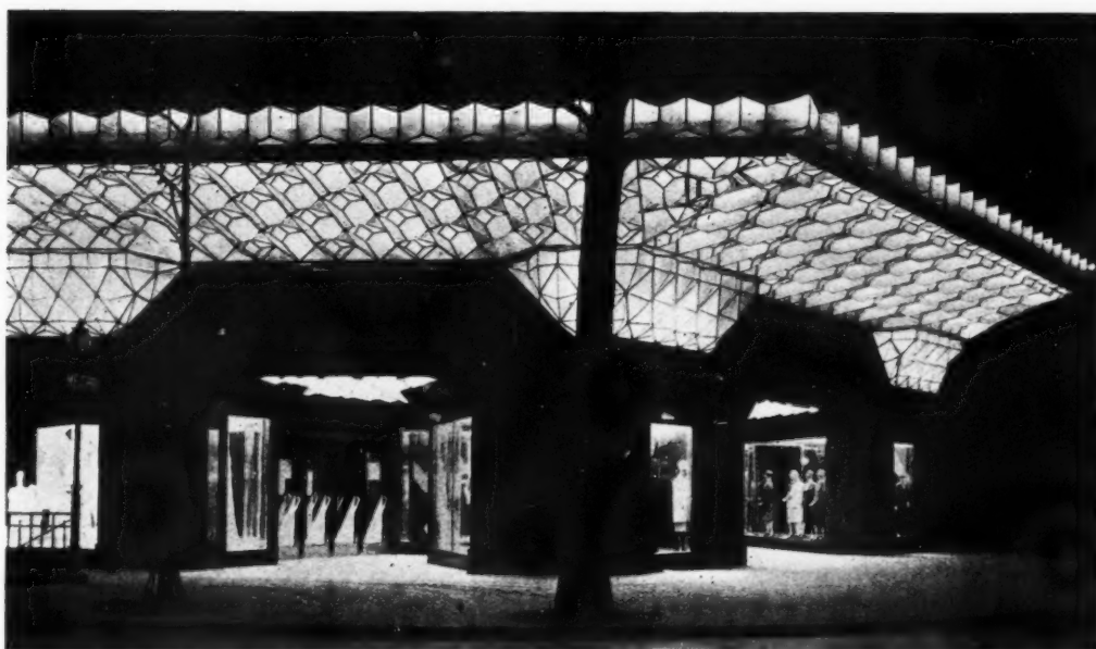
The ground-floor exterior of the Galeries Lafayette, Paris, by M. Chanut, is a remarkable example of the use of glass and indirect lighting on a very large scale. The upper portion of the building is not of recent date. The new ground floor with its many entrances and island showcases is entirely in the modern spirit, and has been almost ruthlessly imposed on the old building.
