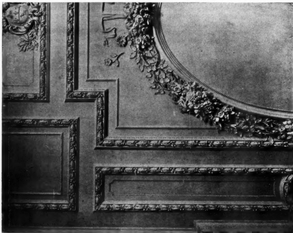
Detail of hand-modelled stucco ceiling done in situ, Acklam Hall, Middlesbrough. By George P. Bankart.
