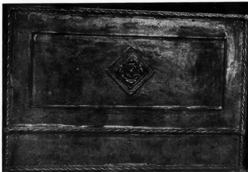
Messrs. Harcourts' Factory, Moseley Street, Birmingham. By James A. Swan. Detail of a cast-iron panel: rough casting before painting, showing screw holes.
