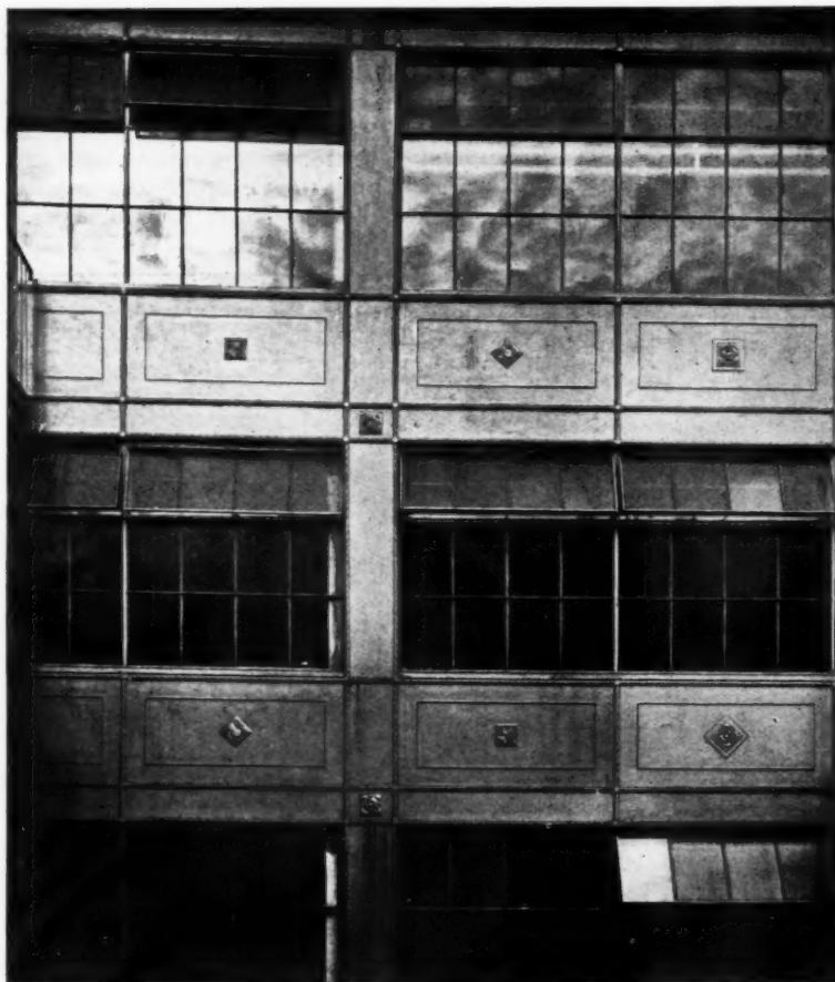
Messrs. Harcourts' Factory, Moseley Street, Birmingham. By James A. Swan. Above, south side of interior court. The whole of the face work is in cast-iron. Below, a detail of the cast-iron fitting to the wall panels.
