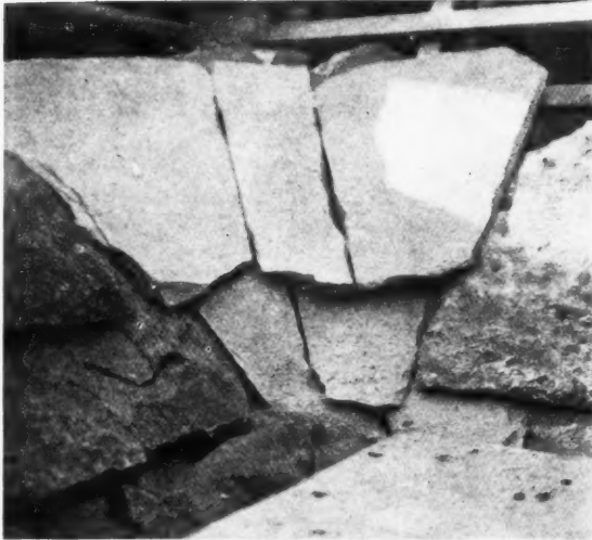
Figure five. Cotswold (Burford) large slates, showing two valley courses.
