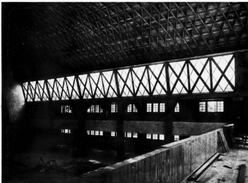
An exhibition hall constructed of wood on the lamella system.
