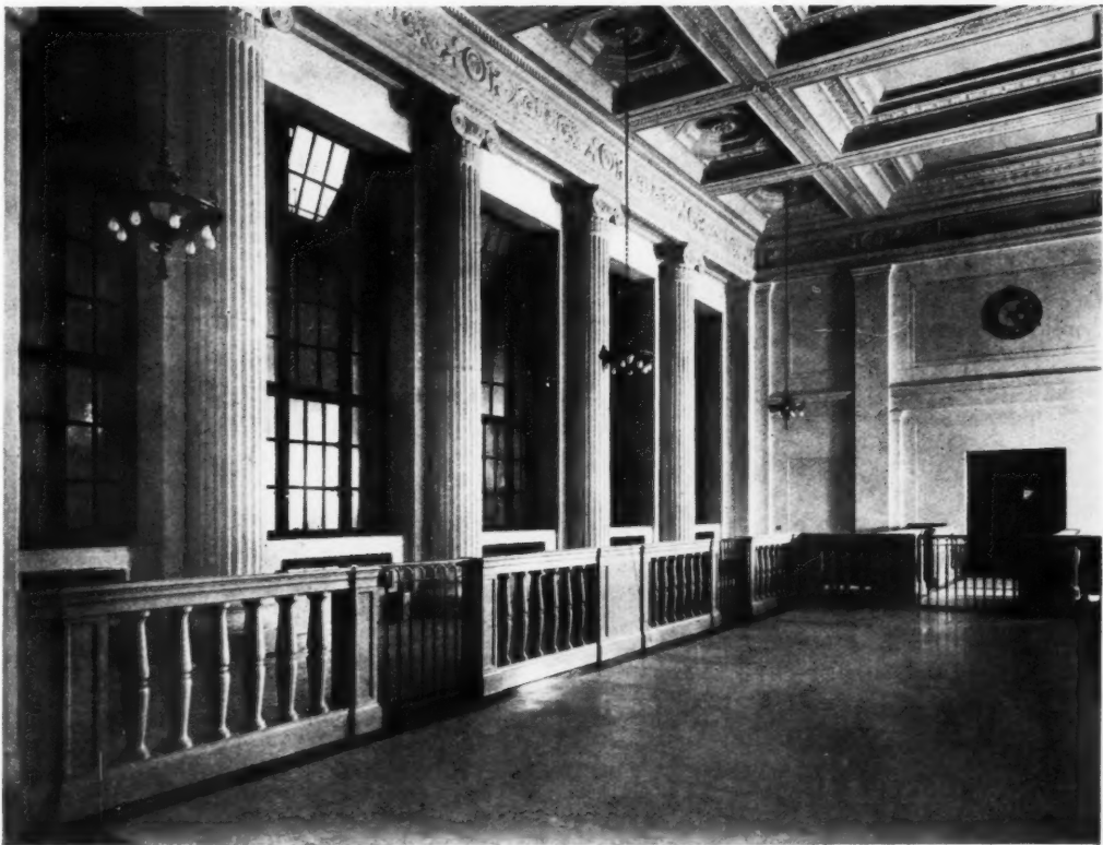
No. 147 Leadenhall Street, E.C. By J. W. O'Connor. Two views of the banking hall from the entrance hall.
