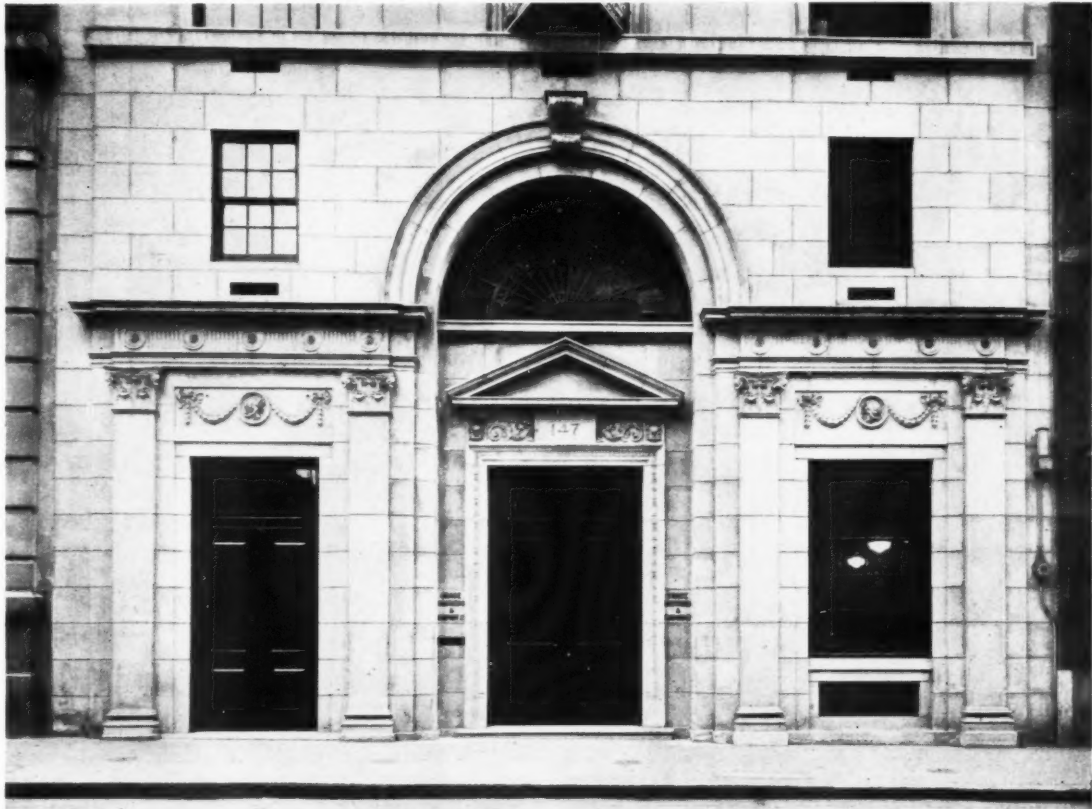
No. 147 Leadenhall Street, E.C. By J. W. O'Connor. Detail of the entrance.
