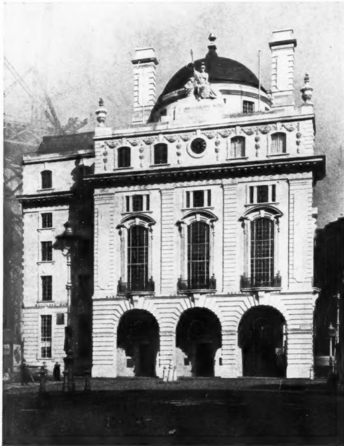
The County Fire Office. Elevation by Sir Reginald Blomfield. Plans by Newton and Woodward.
