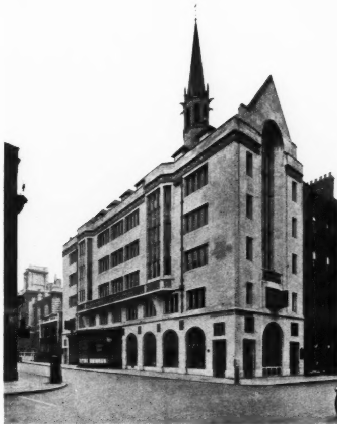
Above, Bond Street Tube Station, London. By Adams, Holden and Pearson. Below, Atkinson's, Bond Street, London. By E. Vincent Harris.
