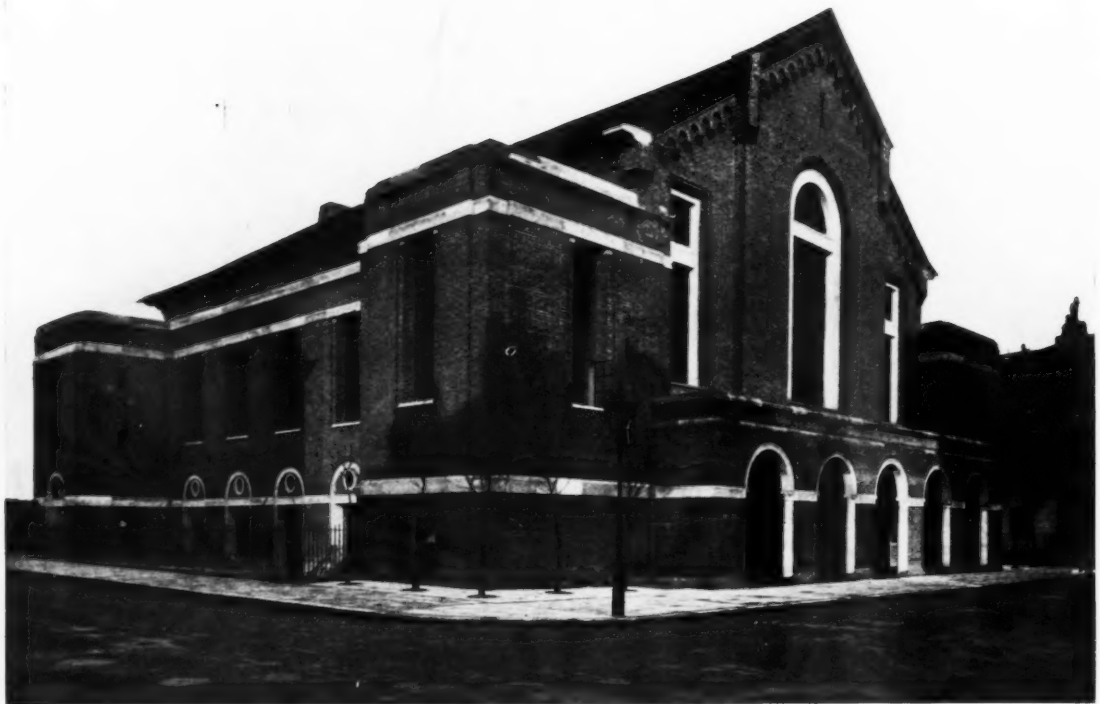
Above, Stockport War Memorial. By Holliday and Agate. Below, Eleventh Church of Christ Scientist, London. By O. P. Milne.
