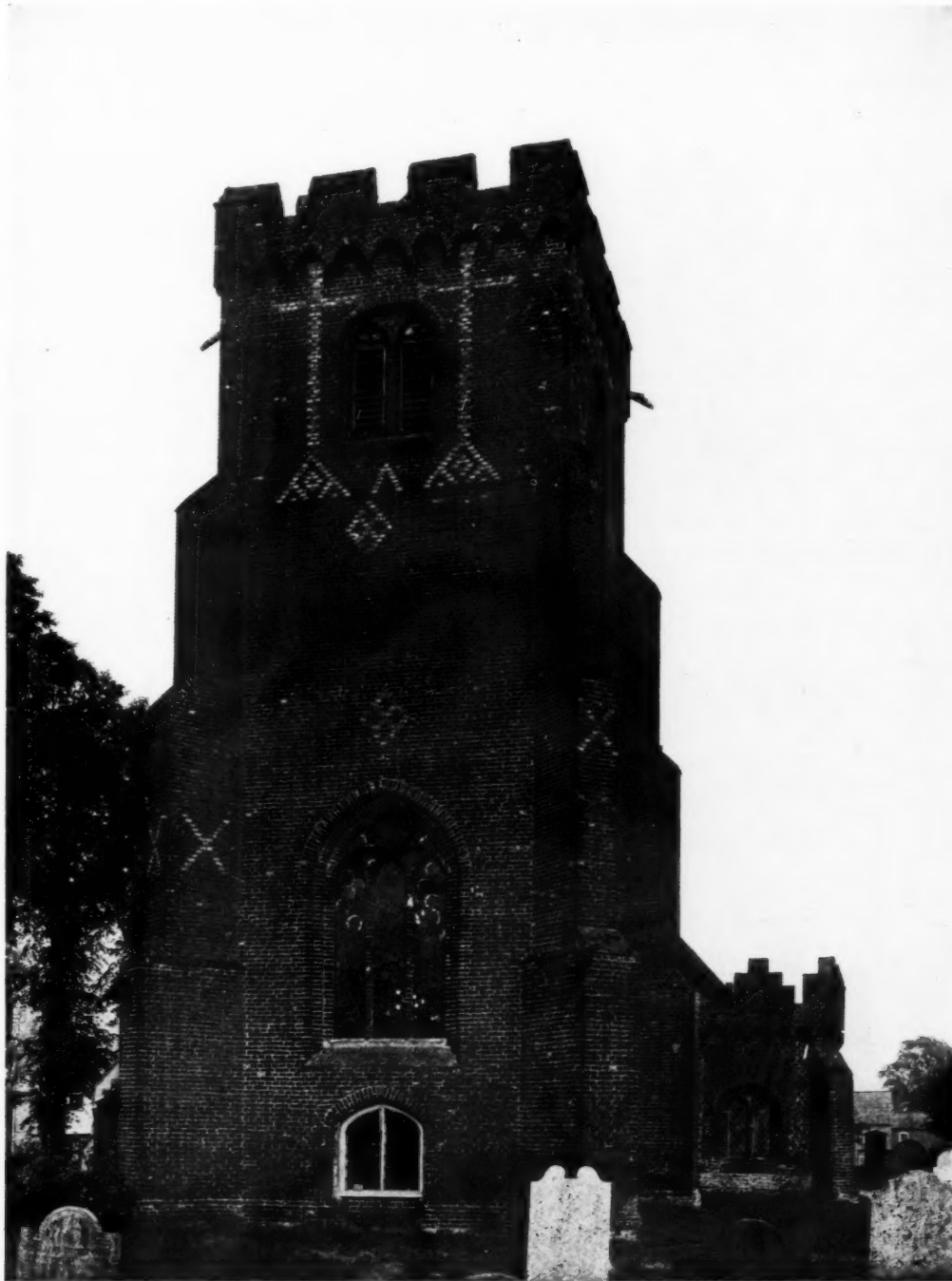
Tudor brickwork, c. 1500. English bond, but somewhat irregular. Such a wall surface shows brick at its best, and compares favourably with the meretricious "neatness" of brickwork in accordance with the "Standard Specification."
