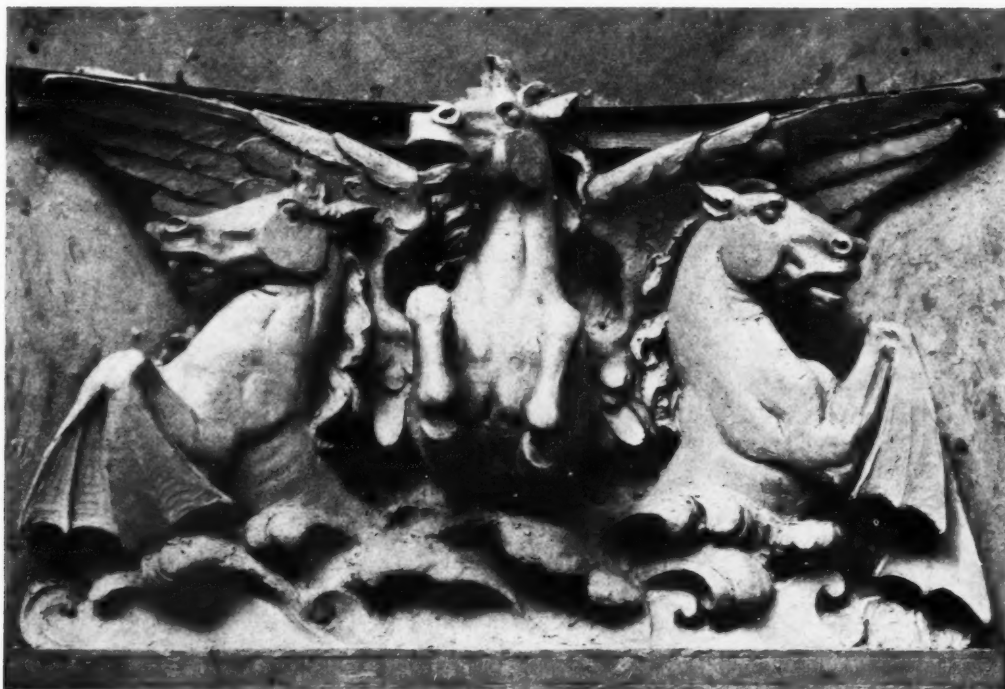
The Royal Mail Steam Packet Company's Building, Cross Street, Manchester. By Grace and Farmer. Detail of carved cast stonework over corner entrance.
