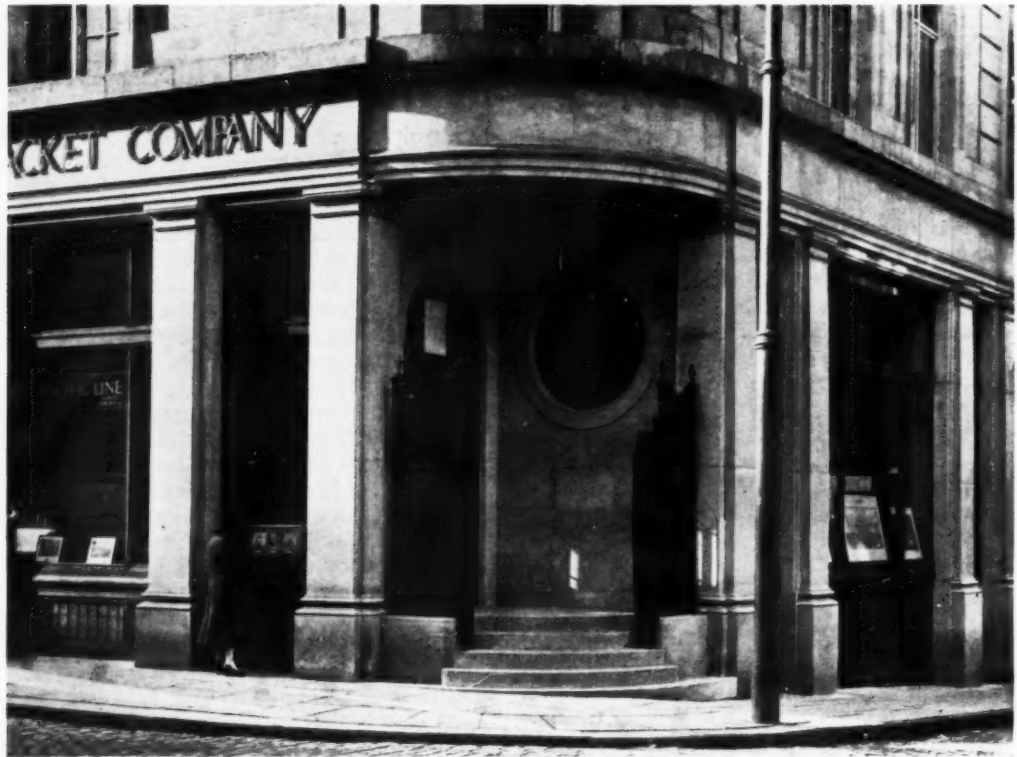
The Royal Mail Steam Packet Company's Building, Cross Street, Manchester. By Grace and Farmer. A detail of the entrance.
