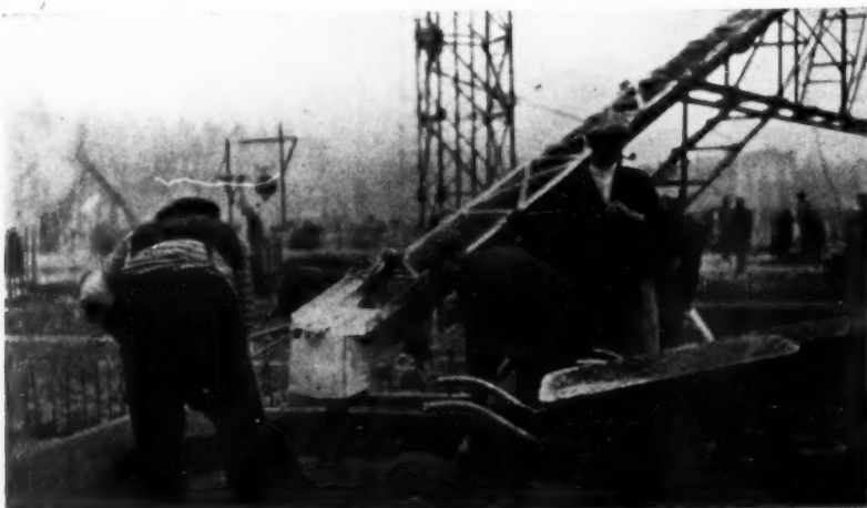
Carreras's new factory, Camden Town. By M. E. and O. H. Collins. Troughs pouring concrete received from tower. There are three towers, each with a radius of 98 ft.
