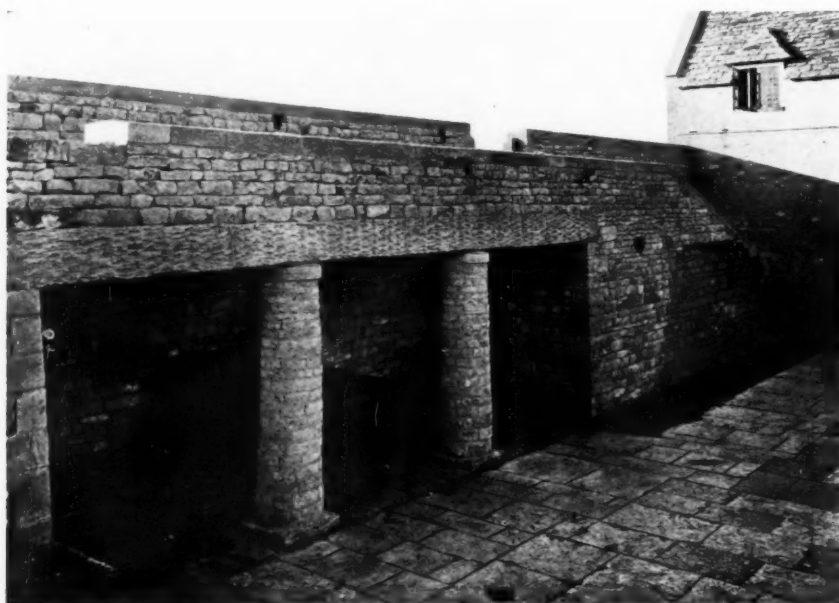
The summer-house. The lintel was made by pouring concrete into shutters lined with specially woven osier hurdles.
