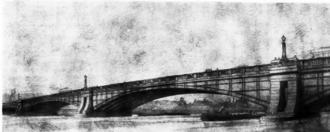
The design for the new Lambeth Bridge. The piers are of stone and the spans of steel. Sir Reginald Blomfield and Mr. C. Topham Forrest, architects. Mr. George Humphreys, engineer.
