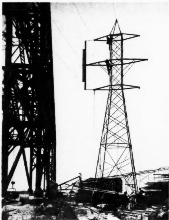
A 110,000-volt tower for the Southern Power Company, U.S.A. This tower, here shown in the construction yard under test, is hardly satisfactory by reason of the top-heavy appearance due to excessive height of the upper parallel portion; the cable arms appear to be too heavy in section and lack bracing which would help to lighten these members.
