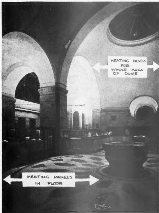
Figure 193. Modern English practice. Concealed panel heating applied to extensive areas of floor and ceiling at the Head Office of Glyn Mills Bank, London.
