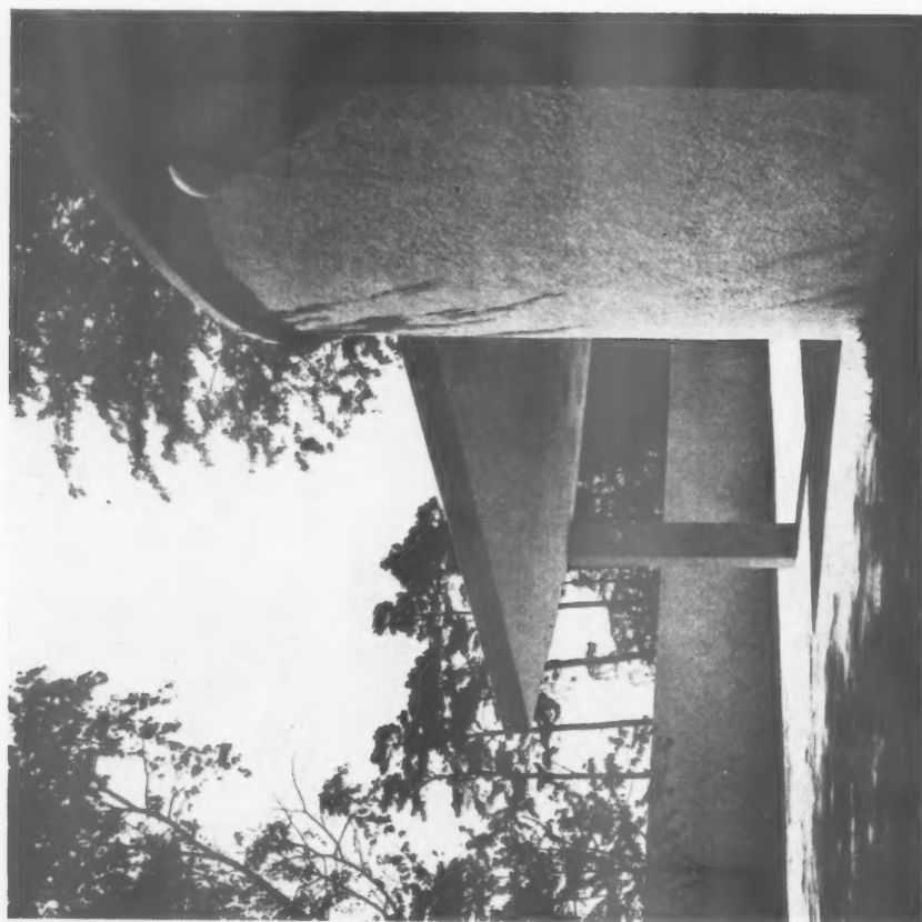
The photographs show : above, a detail of the overhanging day nursery at the south-west end of the building ; right, the north screen wall to the garage approach, showing the R.C. column supporting the washing-space roof.
