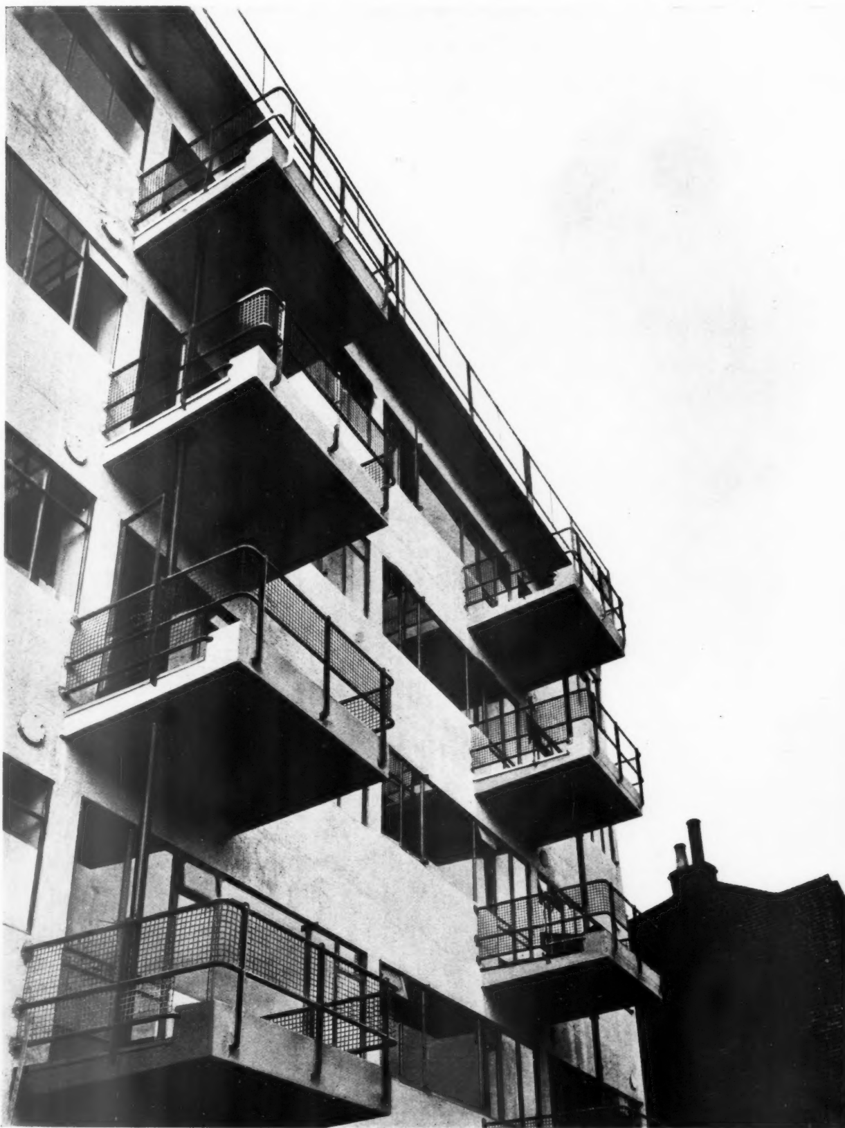
Above is a photograph of a block of working-class flats, showing the cantilevered living room balconies. The front of each balcony is arranged as a flower-box, hence the omission of the wire mesh on the lower half of the railings. Reinforcement details are shown overleaf.
