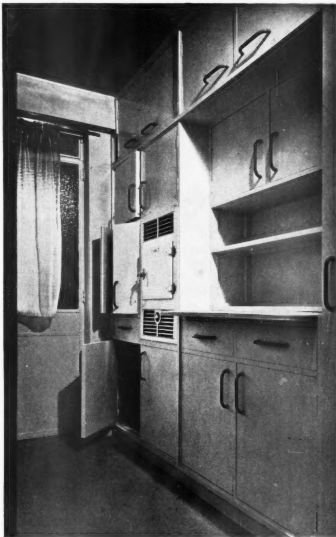
The cupboards illustrated above are built up of deal framing and plywood, painted white. Detail drawings are shown overleaf.
