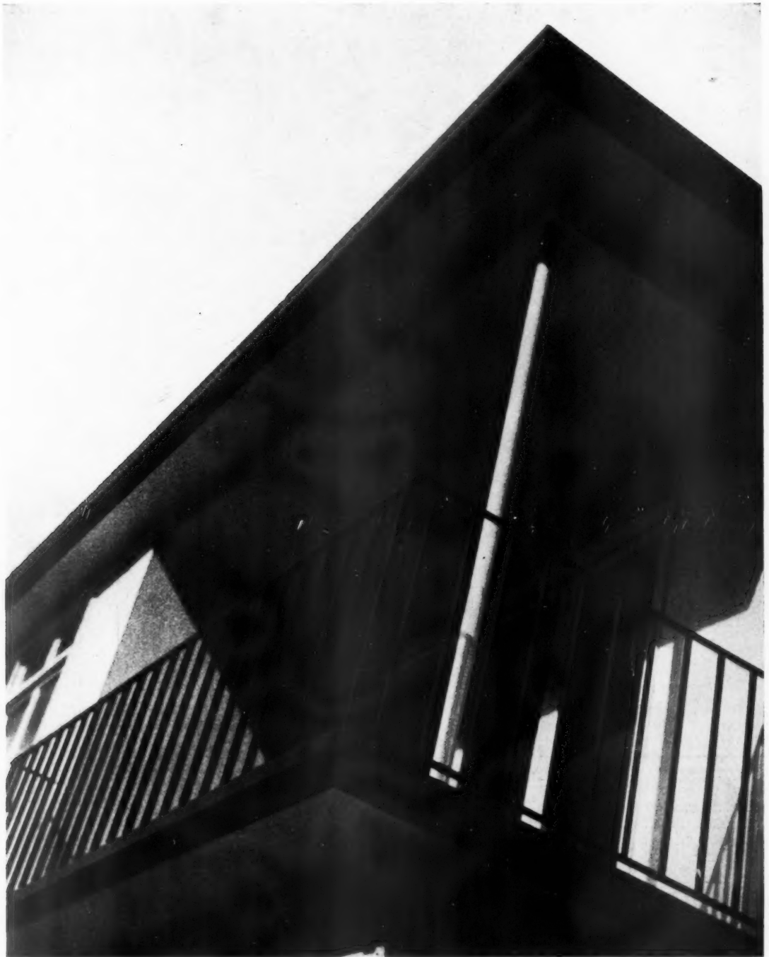
The balcony illustrated above is arranged over a pair of french windows on the ground floor, the bedroom above being set back some 4 ft. at the corner of the building. An axonometric and details are shown overleaf.
