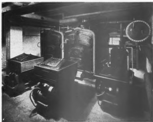
Three typical underfeed type stokers.
