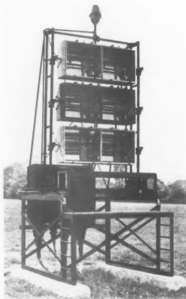
A 3-kilowatt landing floodlight installed at Croydon.
