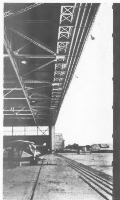
A detail of the hangar illustrated above, showing the roof structure and the arrangement of the sliding doors.
