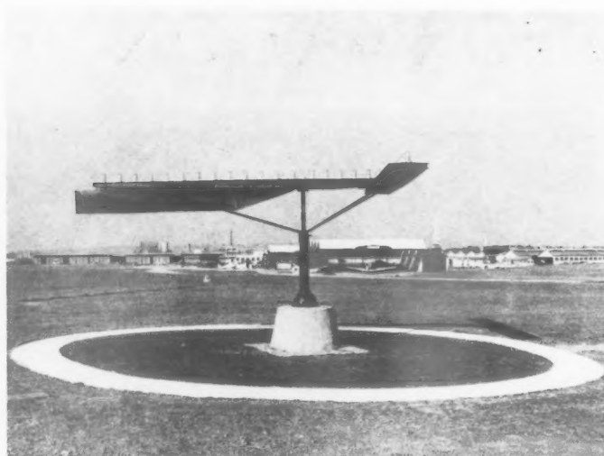
A typical illuminated landing Tee, used to indicate the direction of the wind, and hence the direction of landing. The example shown is at Croydon.
