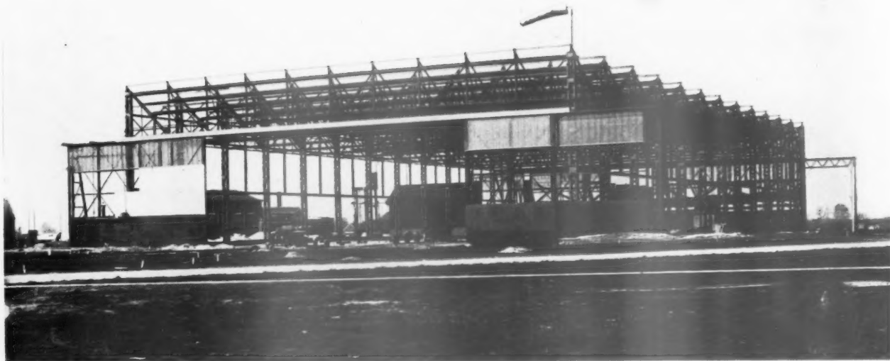
Steel hangar at Mildenhall, with externally sliding doors.
