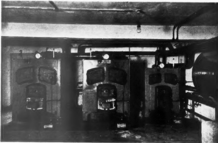
Figure 4: Oil-fired boilers
