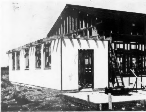
A nursery school of timber and asbestos sheeting. The right-hand photograph shows the light timber frame completed, and on the left the standard 8 ft. by 4 ft. asbestos-cement sheets are being placed in position.
