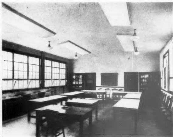
Figure 6: New type of radiator fitted to ceiling of a domestic science room
