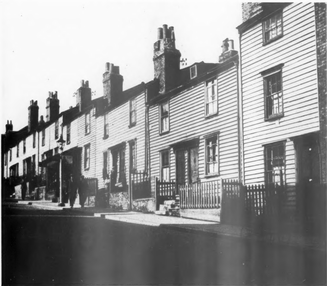
Streets of old English wooden houses are to be seen in Kent, Essex, and sometimes in Norfolk. The above photograph was taken in Kent and shows houses in which brick cores have been used for flues. Up to the early part of the nineteenth century an immense number of the smaller houses and cottages of this county were in this technique of wood construction. From "The Charm of the Timber House."
