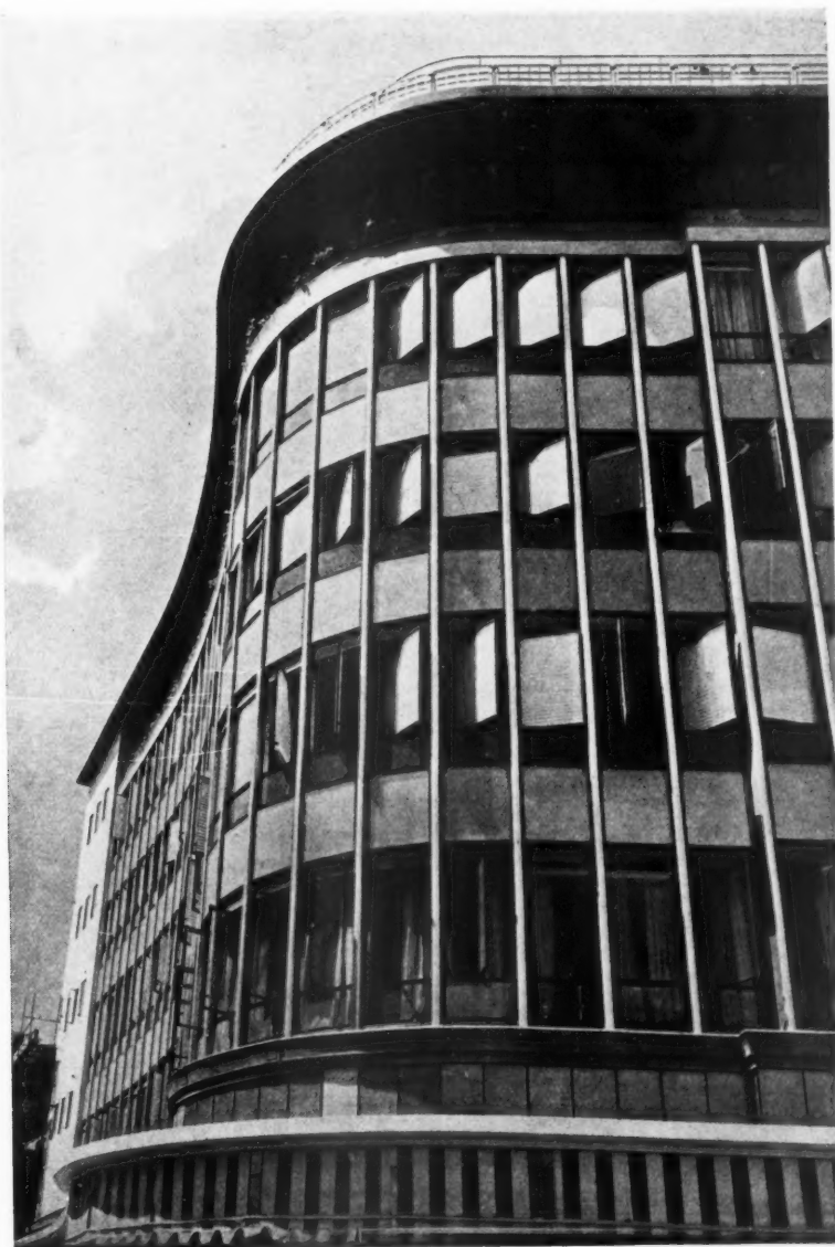
A detail of the upper portion of the façade at the junction of King's Road and Sloane Square. The glass panels between the windows can be opened, and the colour of the building changed by distempering the plaster behind them.
