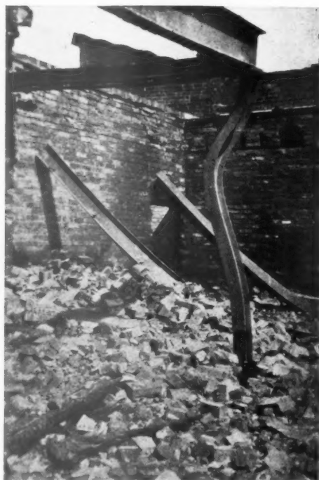
"Both ends fixed"—The result of unprotected steelwork after a fire at Portsmouth.
