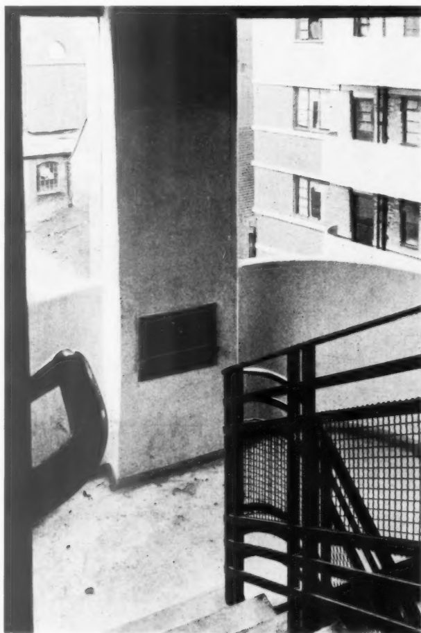
These photographs show the rubbish chute incorporated in the staircases at the Commodore Court Housing Scheme. Rees J. Williams, A.M.Inst.C.E., P.A.S.I., Borough Surveyor. Thomas Sibthorp, P.A.S.I., Architectural Assistant. An axonometric and details are given overleaf.
