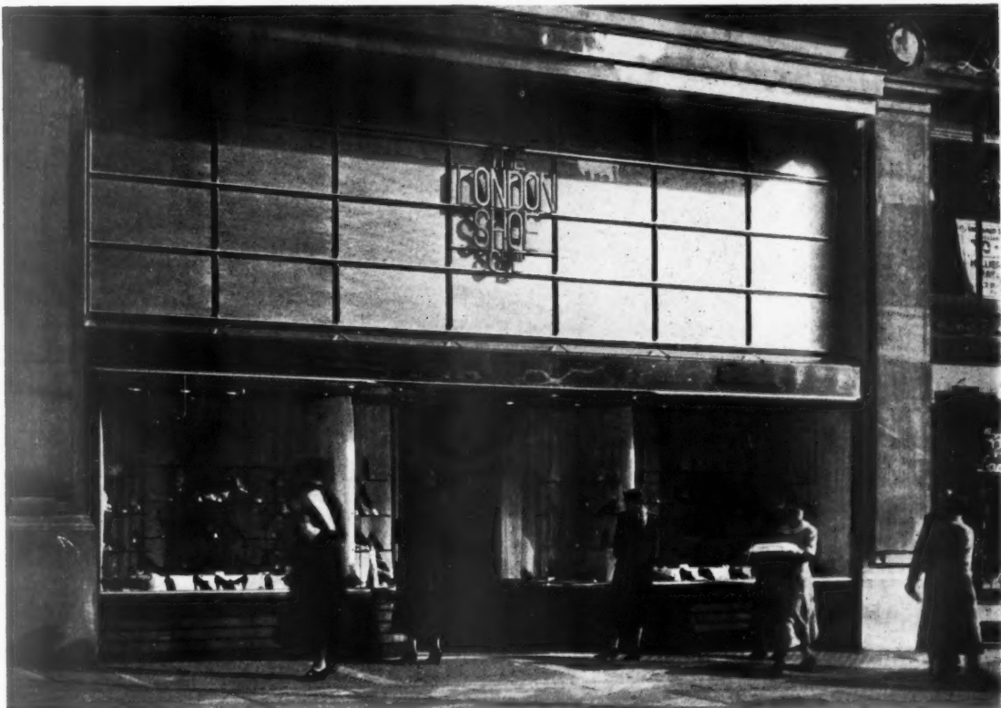
A shoe shop in Regent Street. Thermolux glass has been used for the transome light and the metal work is brass. The glazed brickwork of the stallboard has open joint ventilation slits to the basement.
