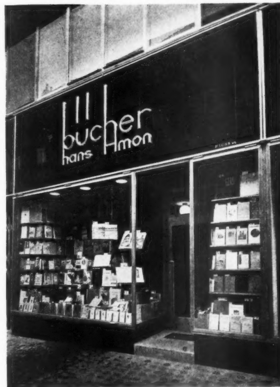
Bookshop in the Herrengasse, Vienna, by Theiss and Jaksch. The front is of polished black marble and the framing, cover strips and lettering of stainless steel.
