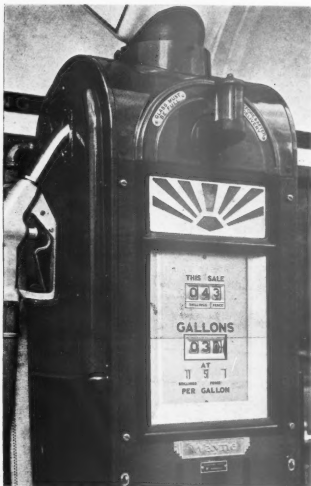
The photographs are : above, head of a petrol pump. The indicator panel shows the price per gallon of the petrol, the number of gallons pumped into the car, and the total cost of the sale ; right, inside the showroom.
