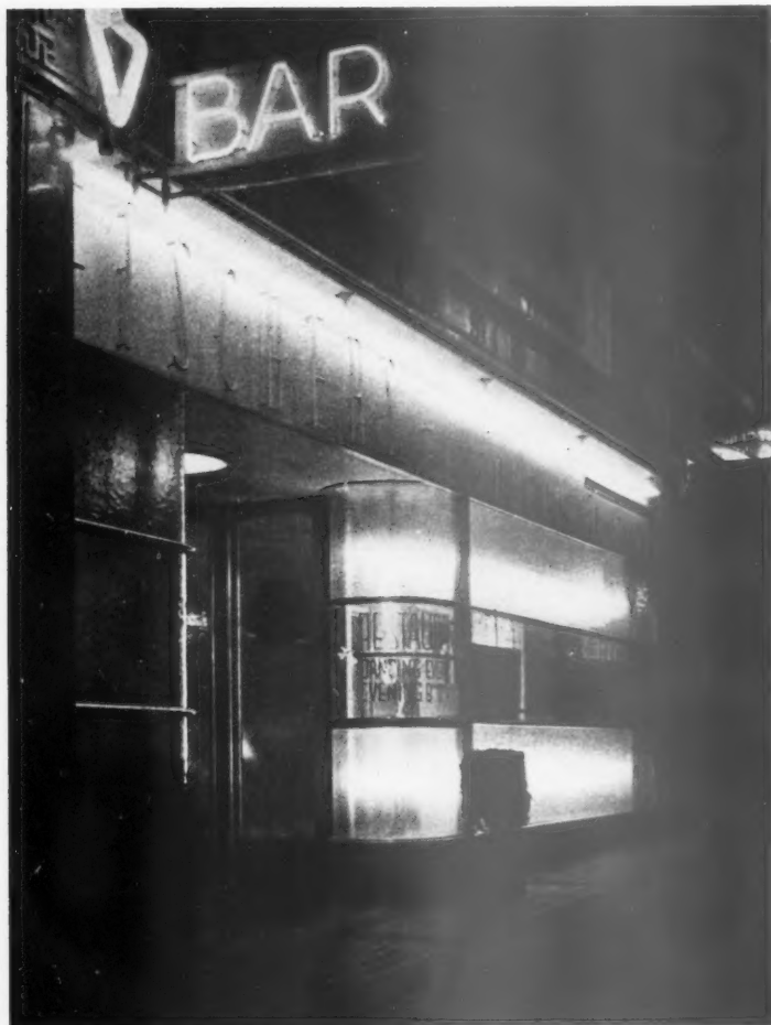
Restaurant by Raymond McGrath showing illumination of fascia and front by Moore tubes. The rough glass breaks up the light, giving an unusual molten effect; the lighting playing a very important part in the design.
