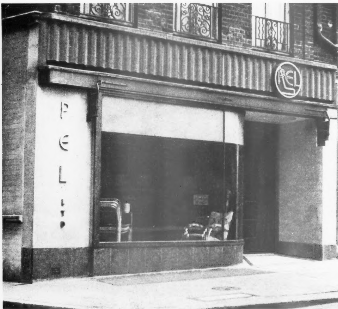
Above : Metal furniture showroom, Henrietta Street, W. Architects, Robertson and Marsh. The materials are Hornton stone plinth with Clipsham stone above. The fascia is made of corrugated asbestos finished with green cement. It is of double construction so as to give "hit and miss" ventilation to the interior, hence the space above the blind box. The metalwork is bronze, and the lettering on the left-hand side is lit by a spotlight above.
