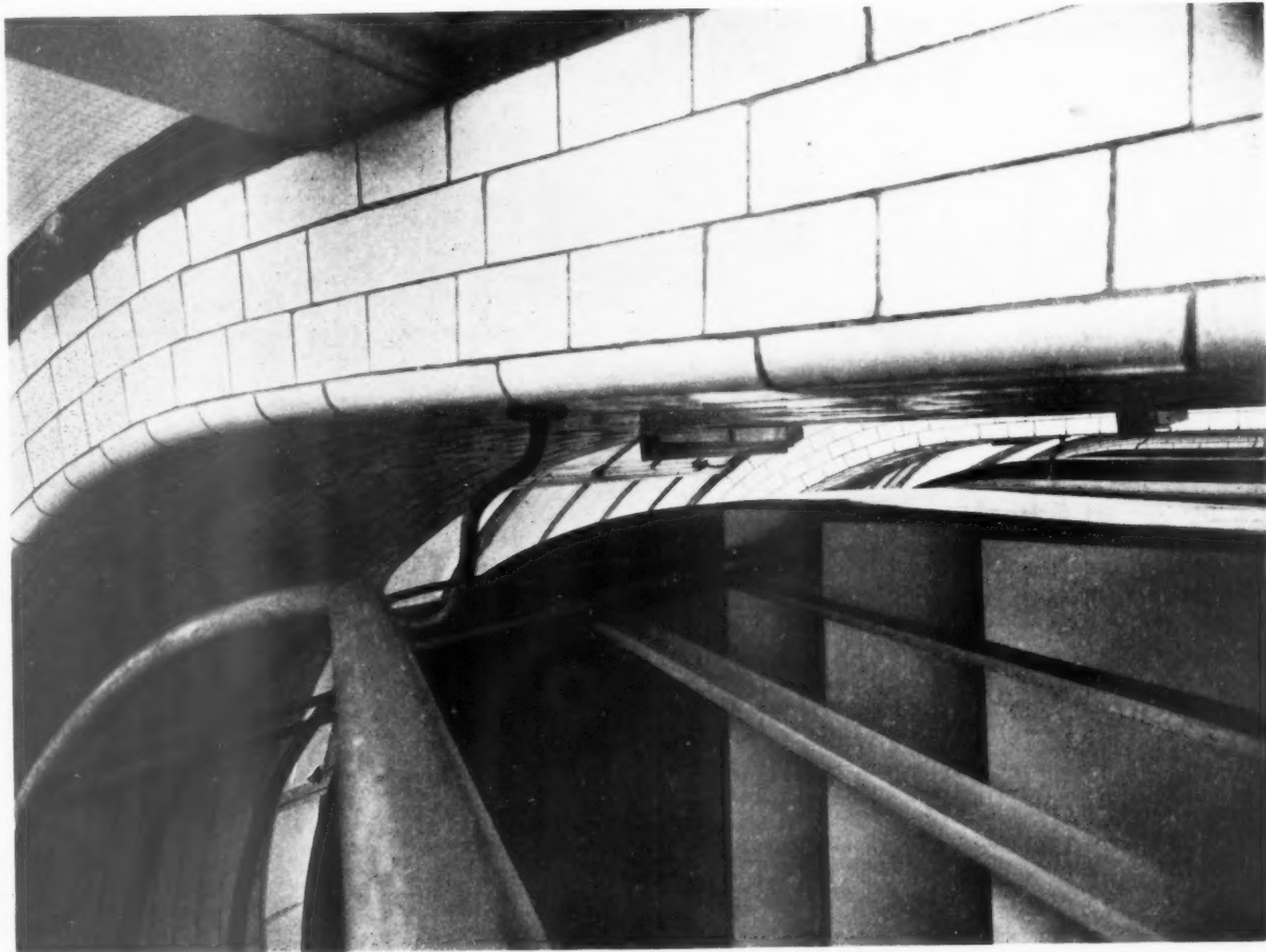
INTERNAL FINISHES —Walls of factory floors are finished in white glazed bricks, with plastered and painted ceilings.
