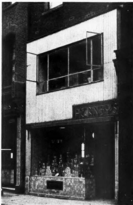
Above : A pleasant arrangement of display windows fitted to show small goods. A large display can be made without the crowded effect so common in shops of this type. The façade is finished in sycamore onyx and bronze.
