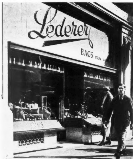
Above : Leather goods shop, Regent Street, London. The character of the shop is gained by the low transome and correspondingly deep fascia. This and the stallboard are in grey opaque glass. The transome is of wood painted green, and the lettering is in bright metal.
