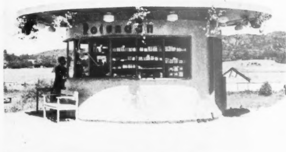
Above: A Swedish kiosk. Chocolates, cigarettes and papers are sold in kiosks of this kind at the side of Swedish roads. The construction is of wooden framing covered with plywood and painted; the metalwork is bronze. The projecting roof and the flowers are attractive features.
