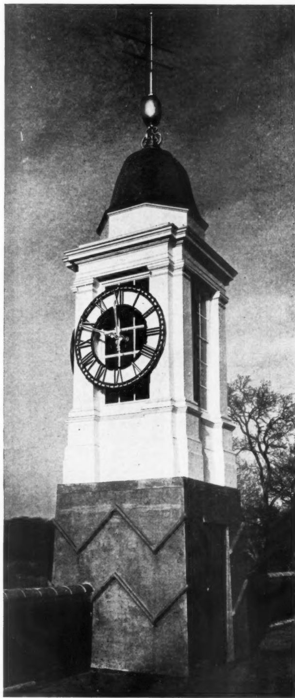
The flèche is constructed in teak framing with tongued and grooved boarding, covered with copper sheeting. The weather vane is in cast bronze. For details see overleaf.
