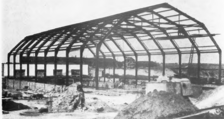
The steel frame for the new Municipal Baths at Thornaby-on-Tees.
