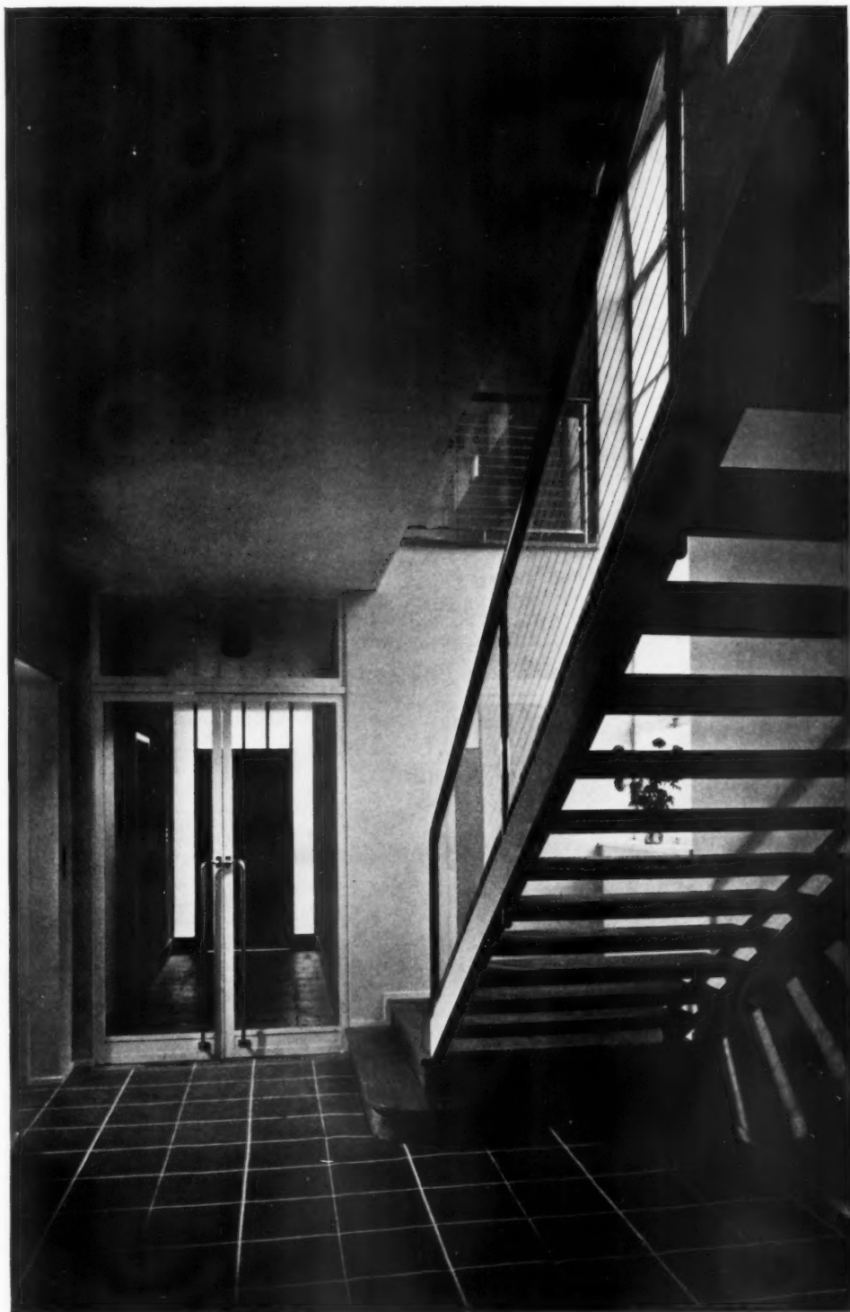
The staircase consists of a series of polished teak treads, supported on metal trays, screwed to the steel channel strings. The balustrade has a polished teak handrail with glass panels carried in a steel channel between steel supports. Details are shown overleaf.
