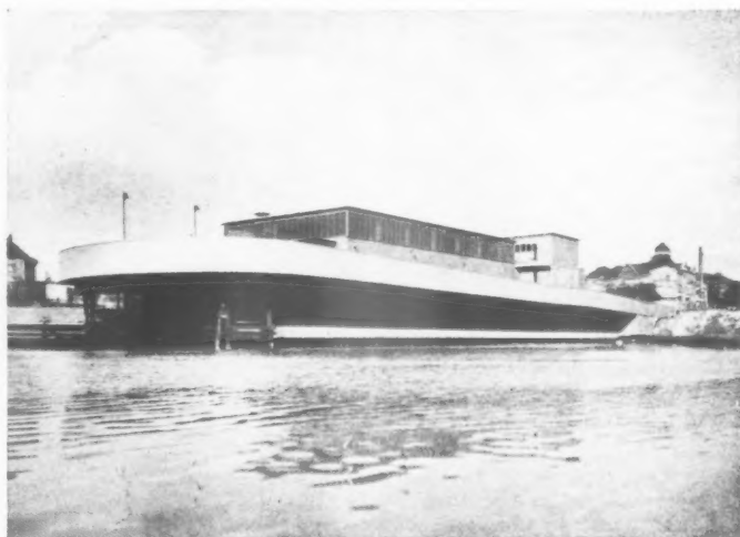
A barge loading station by Paul Baumgarten; goods pass vertically from the barges to the lorry deck above. [From "Bauwelt."]
