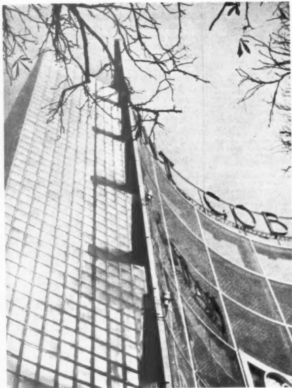
The Saint Gobain glass pavilion at the Paris Exhibition. The sheet glass of the façade contrasts effectively with the glass-brick filling of the return wall. Photo by Norman Westwood.
