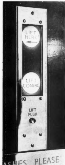
Two photographs showing the control system of the lifts in Athenaeum Court, Piccadilly, described in the accompanying notes.
