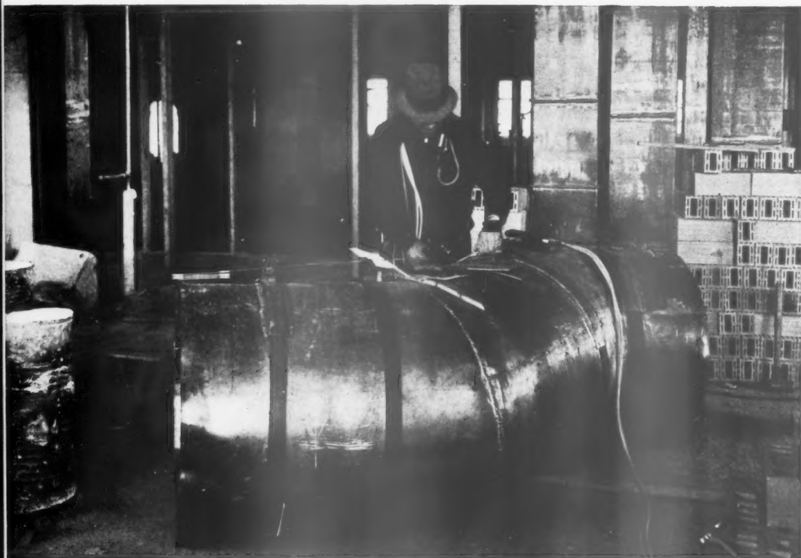
Above. Jointing up the cylindrical duct showing leadburning to joints in the sheet, and also method of supporting the upper side of the duct by lead strips burned to the ducting on top of the steel bands.
