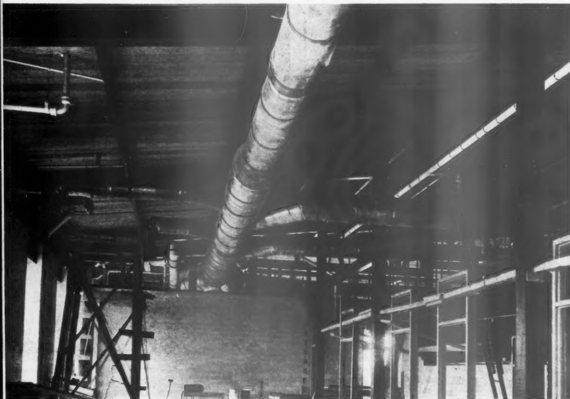
Above. Jointing up the cylindrical duct showing leadburning to joints in the sheet, and also method of supporting the upper side of the duct by lead strips burned to the ducting on top of the steel bands.
