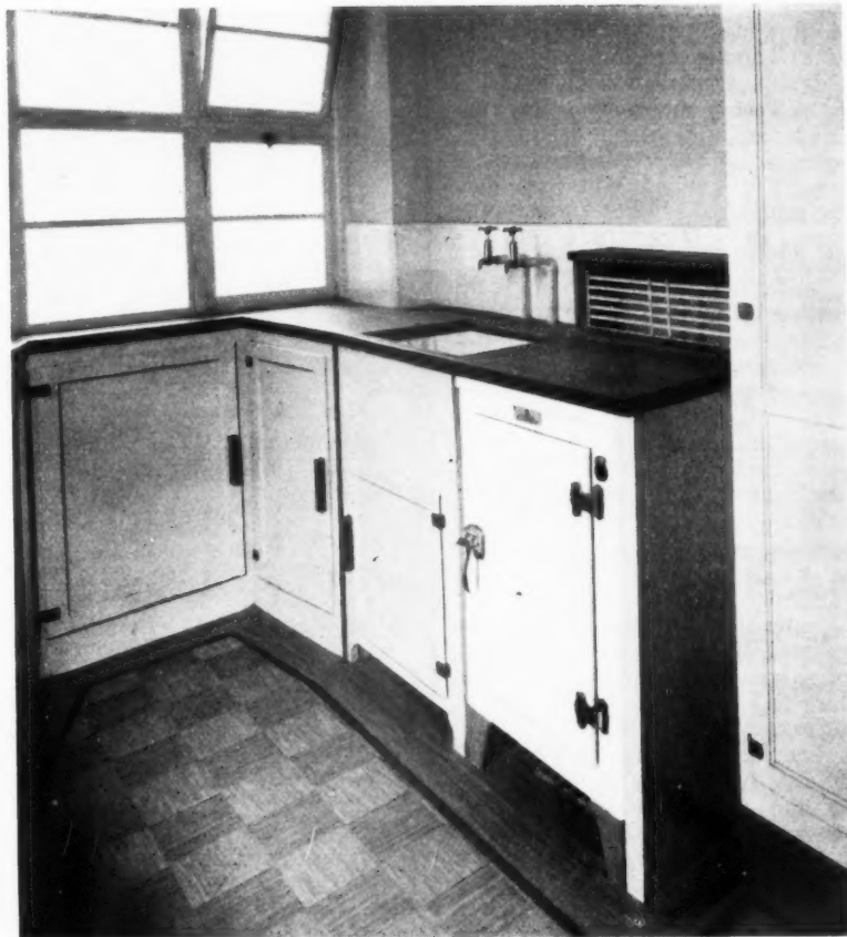
A standard L22 Electrolux gas refrigerator with shortened legs built-in under a draining board. As a standard domestic model has been used, it has been necessary to provide the grille shown above the draining board to provide ventilation. This appears bad practice, for a cursory inspection suggests that water might easily be splashed through the grille.
