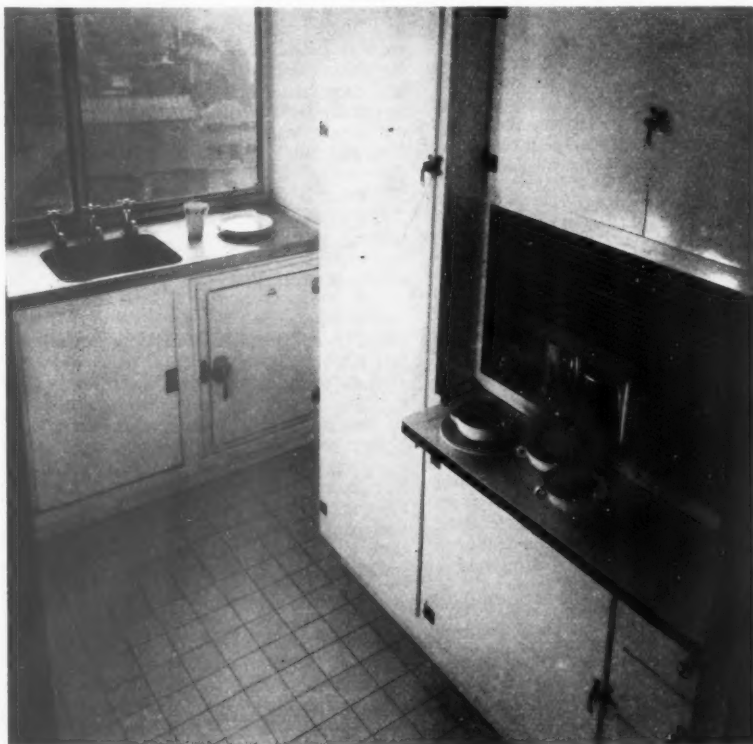
A well-sited central type unit. This type requires no provision whatever for ventilation. This "Frigidaire" model has been incorporated in some large blocks of modern flats, where it is just one of the requirements of the present-day tenant.
