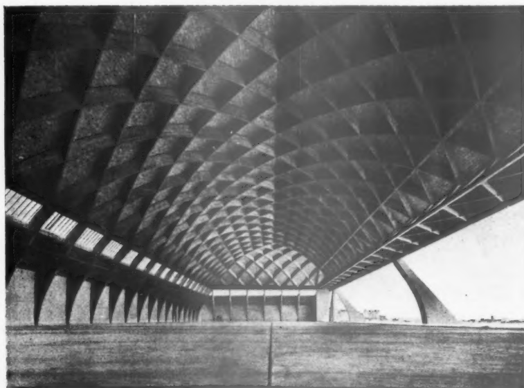
An interesting type of buttressed Lamella hangar construction evolved by Pierluigi Nervi. [From "Architettura."]
