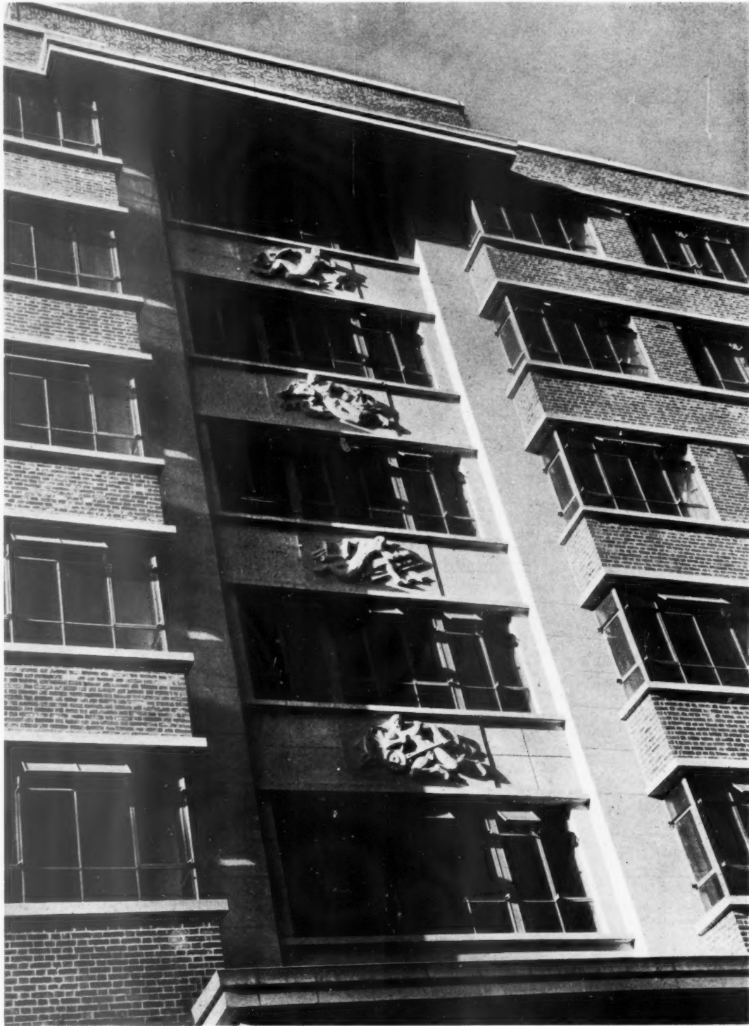
The pre-cast terrazzo slab wall facing and panels above the main entrance to the office block. The panels were cast and finished complete in one piece in the workshops, from the original clay models by Mr. Bainbridge Copnall.
