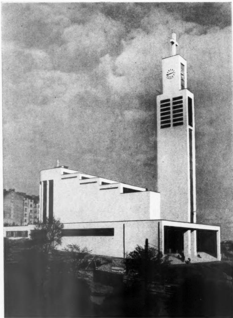
The Church of St. Wenceslas, Prague, by Josef Gocar. The use of reinforced concrete trusses (see section) allows the nave to be free from columns.—[From the "Architectural Record."]
