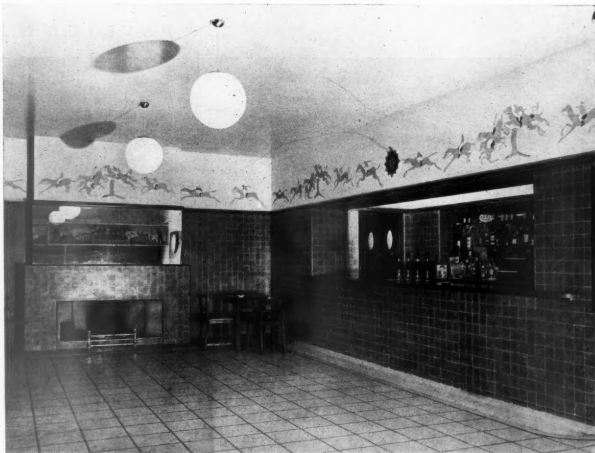
The public bar; the walls are lined with 4-in. brown tiles, eggshell finish, with teak capping and skirting, and counter front in tiles. The painting on the mirrored glass over the fireplace and the decorative frieze above the tiling all round the bar are by Cosmo Clark.
