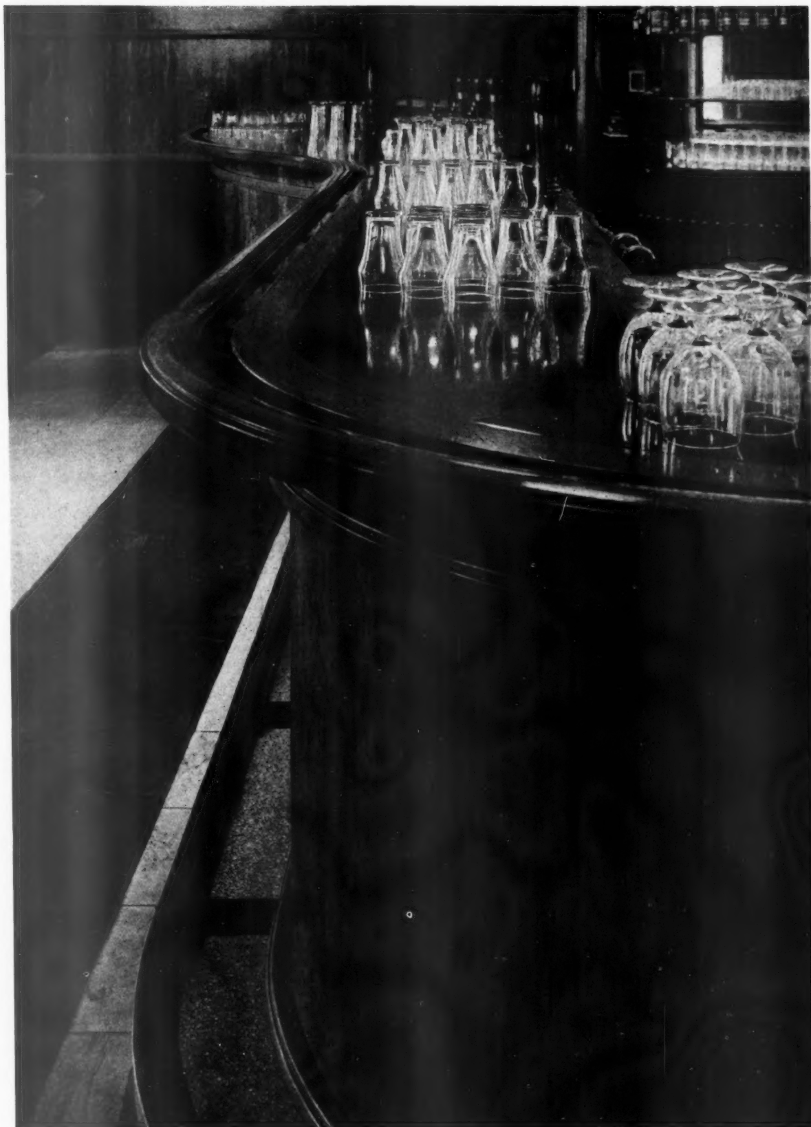
A detail of the counter in the saloon bar. The rail at the top enables the customer to lean against the counter without staining his clothes with beer.
