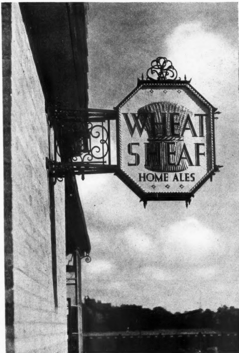
This double-faced sign, on The Wheatsheaf Hotel, at Wolverhampton, consists of two double-hammered wrot-iron plates, each carrying a hand-beaten copper modelled sheaf. The bracket and monogram are in delicately worked wrot-iron, finished grey. The background colour on the plates is cream; the sheaf is picked out in gold and wheat-coloured tones in enamel; the rope surrounding ornament is in gold, and the superimposed lettering is in flame-red enamel. The building upon which the sign hangs was designed by Mr. T. Cecil Howitt, and is illustrated on pages 846-847.
