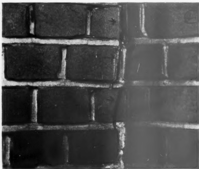
1 and 2 Outside and inside of a bay, showing crack between semi-circular brickwork of bay and main wall of house; and the same crack on the inside face of wall. This house, the JOURNAL was told, has no foundations other than an alleged 4 ins. of site concrete.
