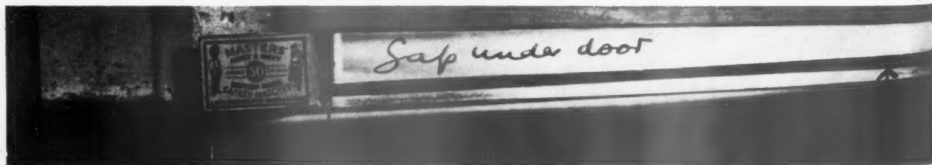
3 A tapering gap under a living-room door. This, the JOURNAL was told, has developed since the house was built.
