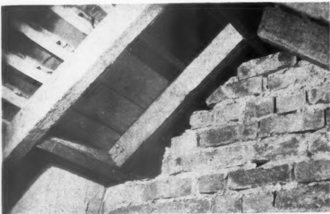
6 Joists, trimmers and lathing continue across a party wall, leaving a 4 in. to 10 in. gap between houses.
