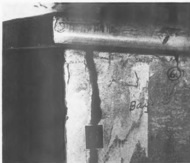
1 and 2 Outside and inside of a bay, showing crack between semi-circular brickwork of bay and main wall of house; and the same crack on the inside face of wall. This house, the JOURNAL was told, has no foundations other than an alleged 4 ins. of site concrete.
