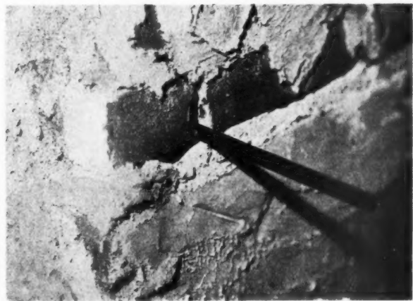
7 Five feet of steel rule has been pushed into an open perpendicular in a chimney breast. Whether it coiled up in the flue or went through into adjoining property is not known.
