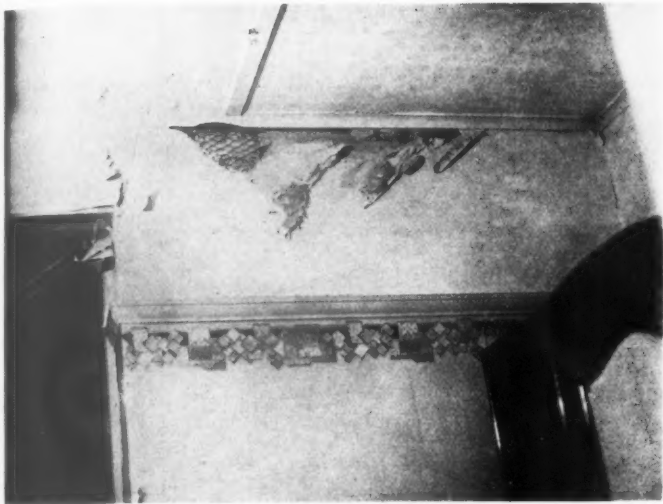
4 Failure of plaster in bedroom. A collection of bits of brick, timber and wire-mesh are exposed.
