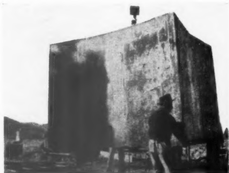
A Los Angeles company has evolved a method of pouring reinforced concrete houses with pipes, services, window frames and interior trim all in place. The photographs show, left, the internal formwork the size of a complete room being placed on the foundation slab; right, the placing of the outer formwork after reinforcement and services have been installed. [From the "Architectural Forum."]
