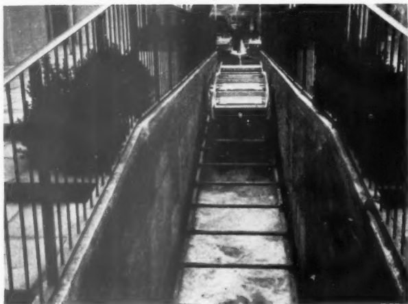
The waterway in which visitors are pushed round the Zurich Exhibition in small boats. The photograph shows the rollers over which the boats slide down slopes while the water runs down at a lower level.
